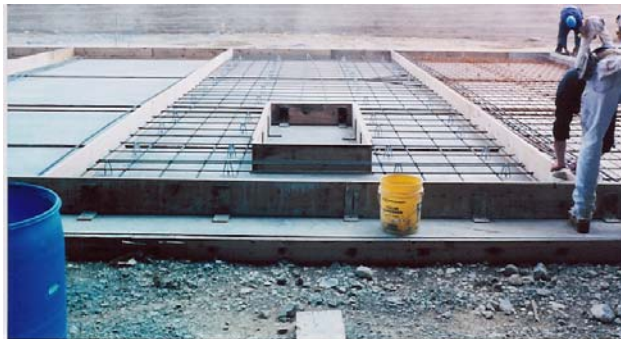
1013 1014 1015 1016 1017 1018 1019 1020 1021 1022 1023 1024 1025 1026 1027 1028 WWR Sheets for Tilt-up Wall Panels
