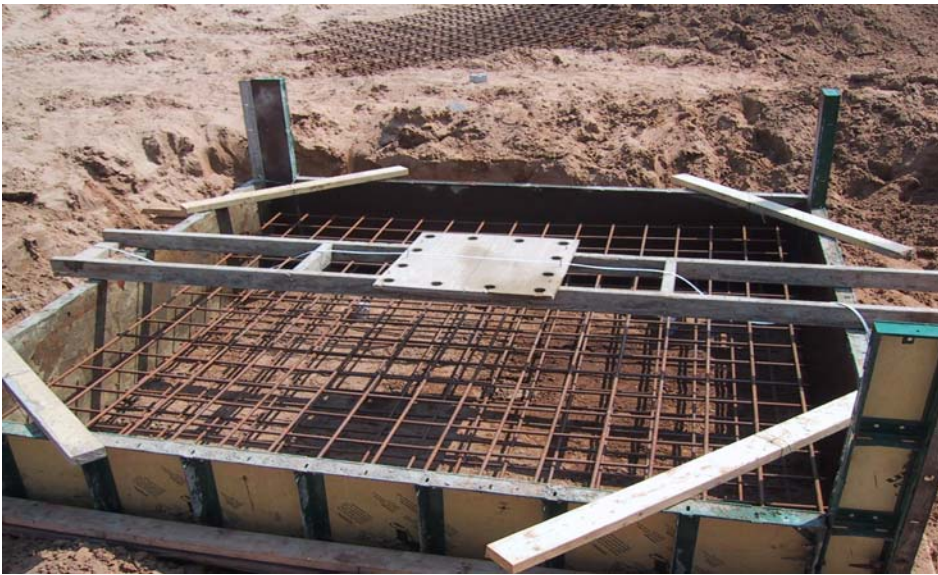
WWR in Spread Footing for Ice Mountain Project
