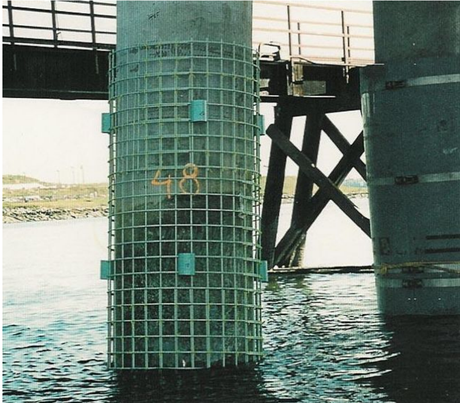
Rolled WWR Column Retrofit for Rykers Island Pier
