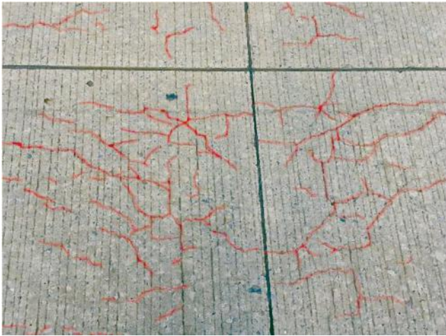
Fig. 1—Concrete pavement D-cracking, Interstate 49.
