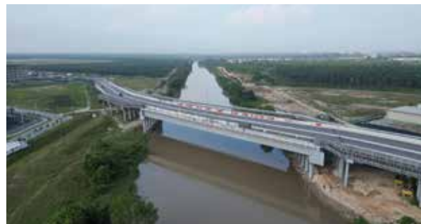
BRIDGES - First Place 105 m Span Ultra-High-Performance Concrete (UHPC) Composite Bridge, Kuala Langat District, Selangor, Malaysia
