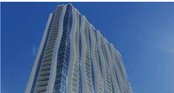
HIGH-RISE STRUCTURES - First Place Kō'ūla, Honolulu, HI, USA
