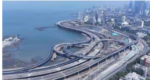
INFRASTRUCTURE - First Place Mumbai Coastal Road, Mumbai, Maharashtra, India
