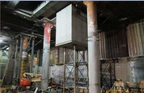
Hub room slab on micropiles to support track equipment. Couplers used to connect to new slab.
