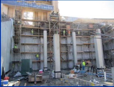
Shotcrete Operation on Historic Wall
