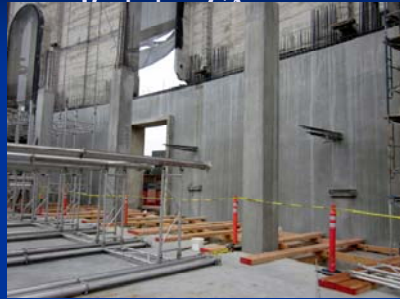
Finished Shotcrete Historic Wall
