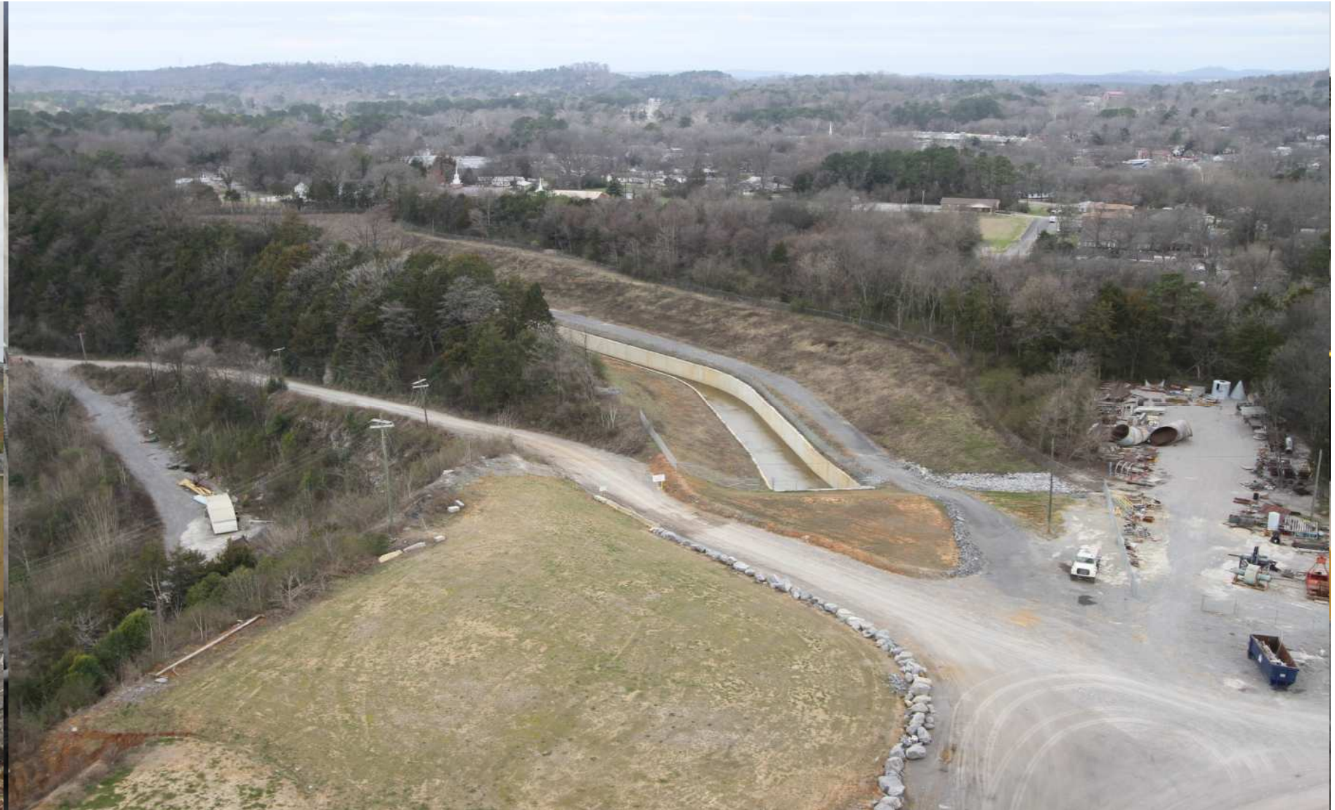
100 Year Old Cement Plant with Sustainable cements Gary Knight 4/15/13
