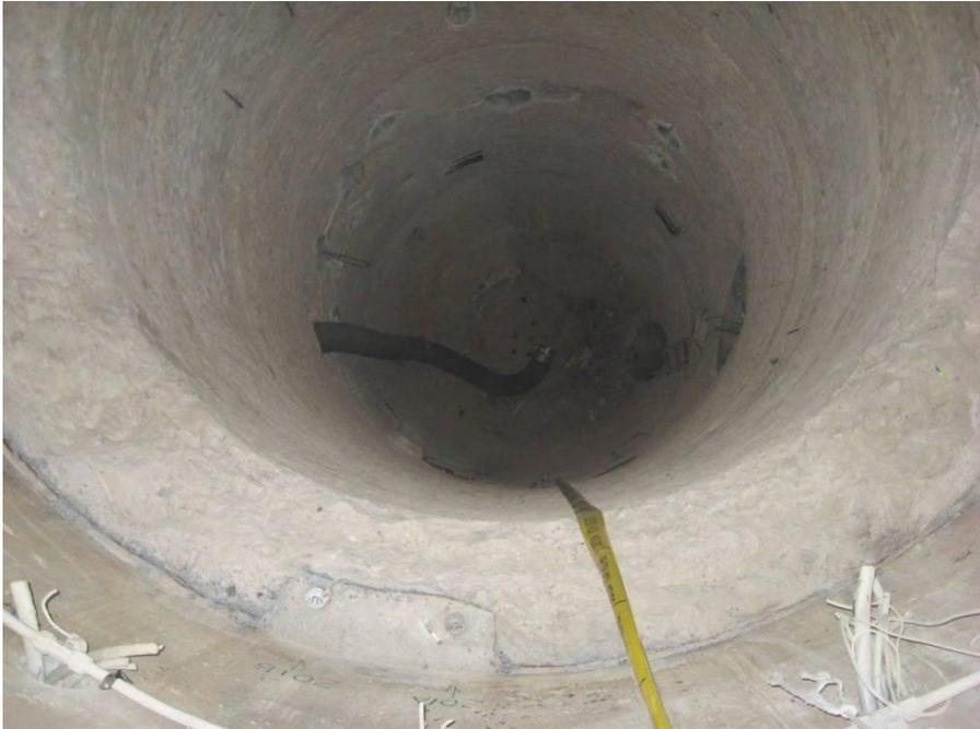
Reactor cavity concrete may see  $> 10^{20}$  n/cm<sup>2</sup> during the period of Long Term Operation, which is beyond the design basis.
