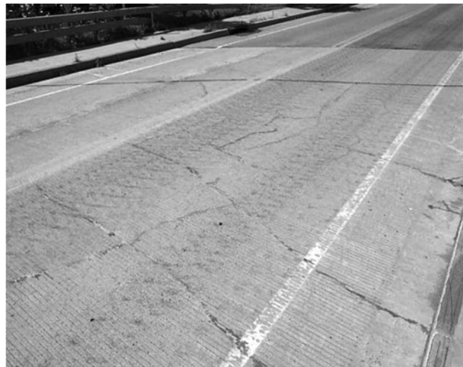
Fig. 1—Methacrylate flood coats are well-suited to concrete slabs that have a large number of random cracks but no evidence of steel corrosion or AAR.
