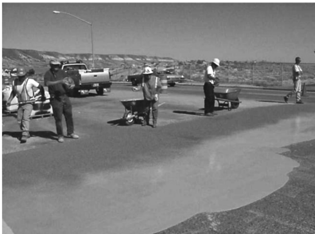
Fig. 4—Aggregate should be broadcast over the surface before the resin becomes tacky but at least 20 minutes after applying the final coat.
