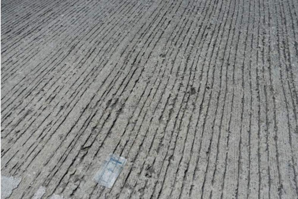
**Fig. 2**—Freeze-thaw damage and aggregate pop-outs on IN-IC-HPC-2
