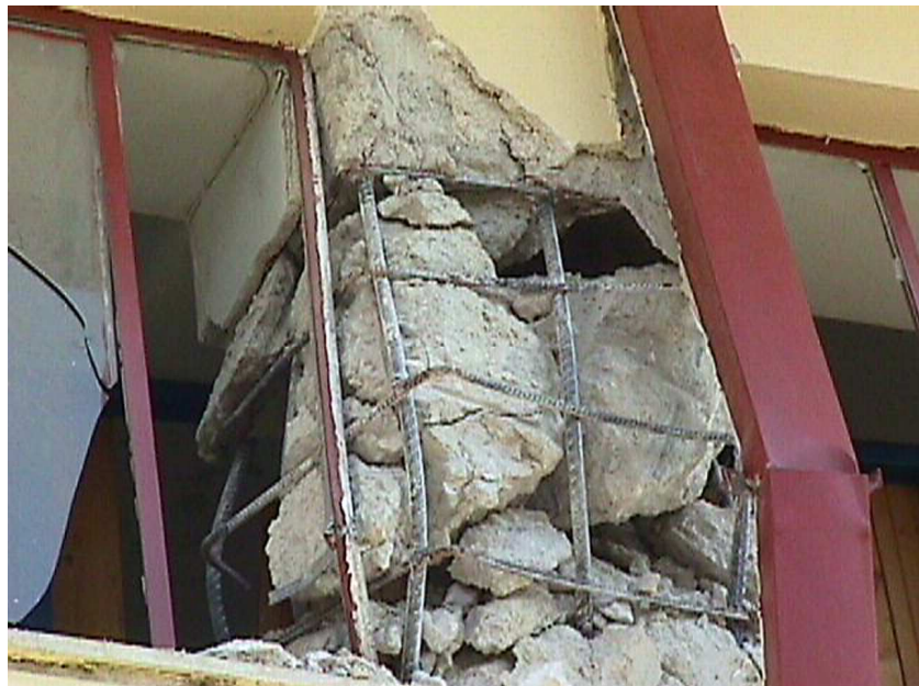
Failure of a column dimensioned according to old regulations that required a peripheral stirrup with its end bent in 90° instead of 135° (45°).
