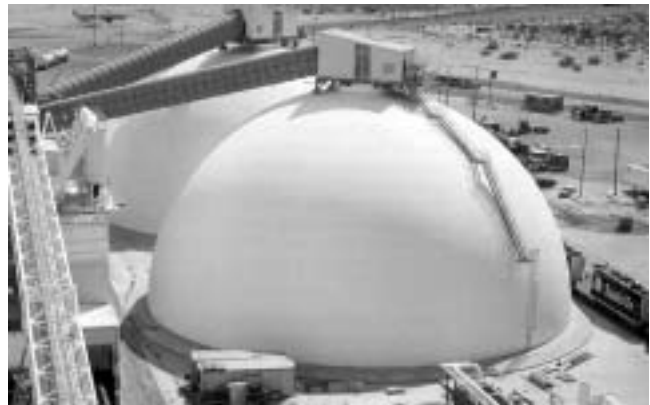
Fig. 1.3—U.S. Borax and Chemical Co., Boron, Calif.: two 20,000 ton (18,000 tonne) borax storage domes, 150 x 79 ft (45.7 x 24.1 m).
