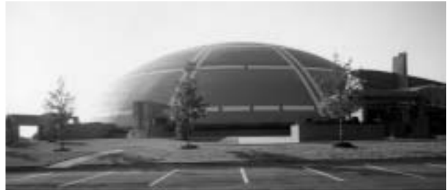
Fig. 1.1—Faith Chapel Christian Center, Birmingham, Ala.: 280 ft (85.35 m) diameter and 72 ft (22 m) tall that includes a 3200-seat sanctuary, classrooms, and an administration building.
