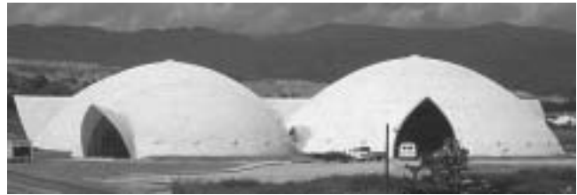
Fig. 1.2—Price City Works Complex, Price, Utah. Four domes: 130 x 43 ft (40 x 13.1 m) fire station; 130 x 43 ft (40 x 13.1 m) storage facility; 130 x 43 ft (40 x 13.1 m) maintenance shop; and 90 x 40 ft (27 x 12.2 m) office and administration building.
