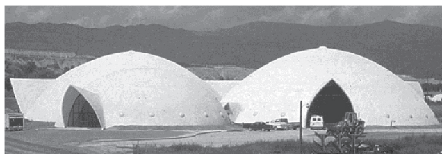
Fig. 1.2—Price City Works Complex, Price, UT. Four domes: 130 x 43 ft (40 x 13.1 m) fire station; 130 x 43 ft (40 x 13.1 m) storage facility; 130 x 43 ft (40 x 13.1 m) maintenance shop; and 90 x 40 ft (27 x 12.2 m) office and administration building.
