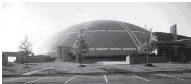
Fig. 1.1—Faith Chapel Christian Center, Birmingham, AL: 280 ft (85.4 m) diameter and 72 ft (22 m) tall, which includes a 3200-seat sanctuary, classrooms, and an administration building.
