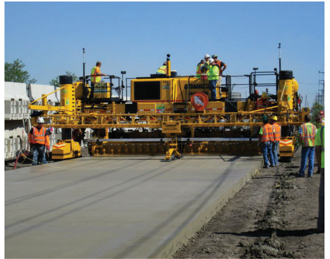
Fig. 3.2.4a—Slipform paver (courtesy of GOMACO Corp.).
