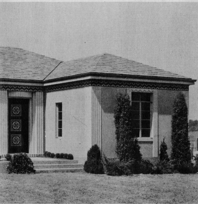
No. 1 Was Built with Prefabricated Walls of Earley Mosaic Combined to Put Enduring Beauty into a Modest Home.
