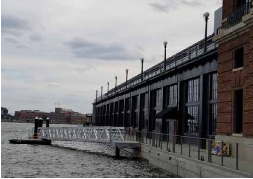
Recreation Pier Hotel – Pier and Bulkhead Restoration
