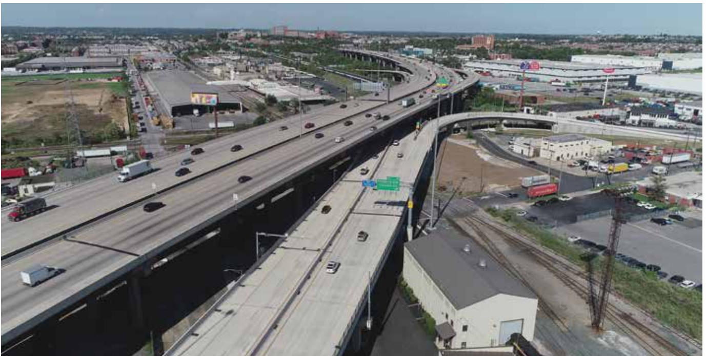
I-895 Bridge Project
