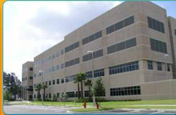
**A** state-of-the-art treatment and research facility, M2Gen is the result of a partnership between Moffitt and drug maker Merck & Co. The exterior features three-colored architectural precast concrete in 247 panels covering 36,600 ft<sup>2</sup>. The chemically retarded exposed aggregate finish was expressed with a medium abrasive blast. Architect: Reynolds, Smith & Hills, Inc. Contractor: Skanska USA.
