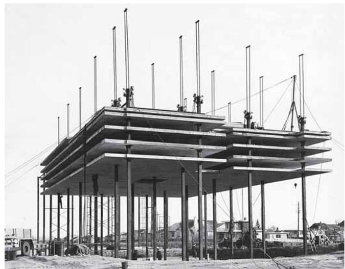
The lift-slab method of construction featured roof and floor slabs that were cast on a base slab with a separating membrane between slabs. Powerful jacks seated on columns raised the slabs to their final position where structural connections between slabs and columns were made.
