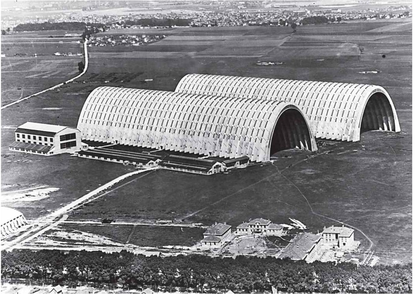
One of the earliest applications of mechanical vibration in placing concrete was that used in building the dirigible hangars at Orly, France, 1921-1924. Utilizing a system of corrugated arches—40 corrugations 10 to 18 ft (3 to 6 m) deep—the hangars had a span of about 295 ft (90 m), a rise of about 195 ft (59 m), and were approximately 984 ft (300 m) long. Engineer: E. Freyssinet. Contractor: Entreprises Limousin.
