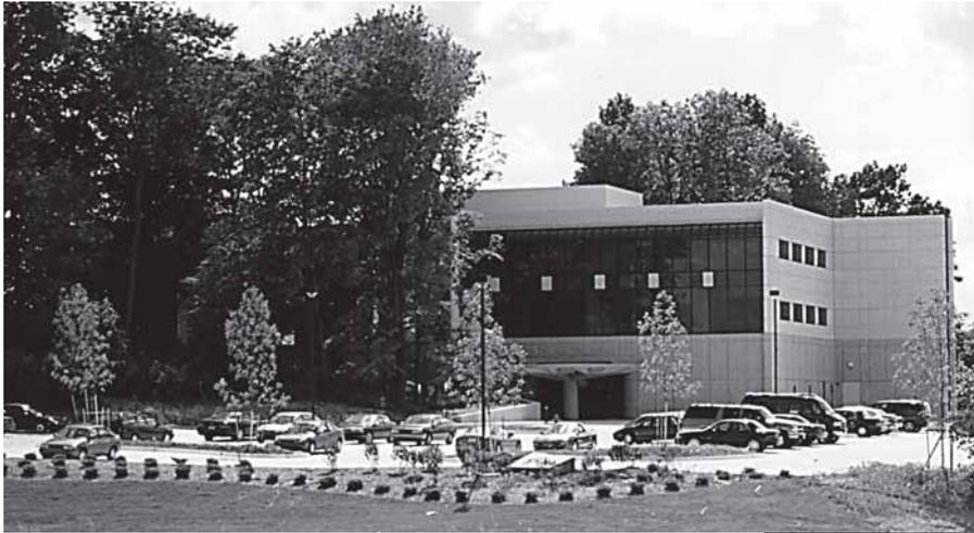
ACI moved into its new headquarters in Farmington Hills, MI, in 1996. The 47,000 ft<sup>2</sup> (4370 m<sup>2</sup>) facility was designed to meet ACI needs through the year 2030. The building is a combination of cast-in-place and precast concrete framing, along with exterior architectural precast wall panels. Inset: A latticework of beams cantilevered from a concrete column formed a semicircular canopy for the main entrance.
