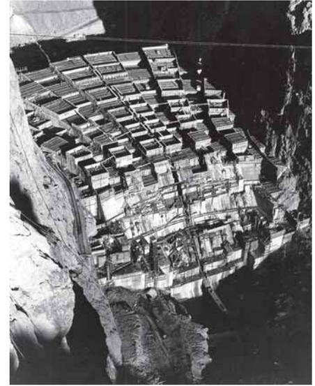
Hoover Dam was the first modern mega project—the greatest dam constructed in its day. For nearly two years, every day, around the clock, a bucket of concrete was dumped into a form every 60 seconds. The dam was raised to 726 ft (221 m) by placing and cooling concrete in 230 massive blocks (December 1933 photo).
