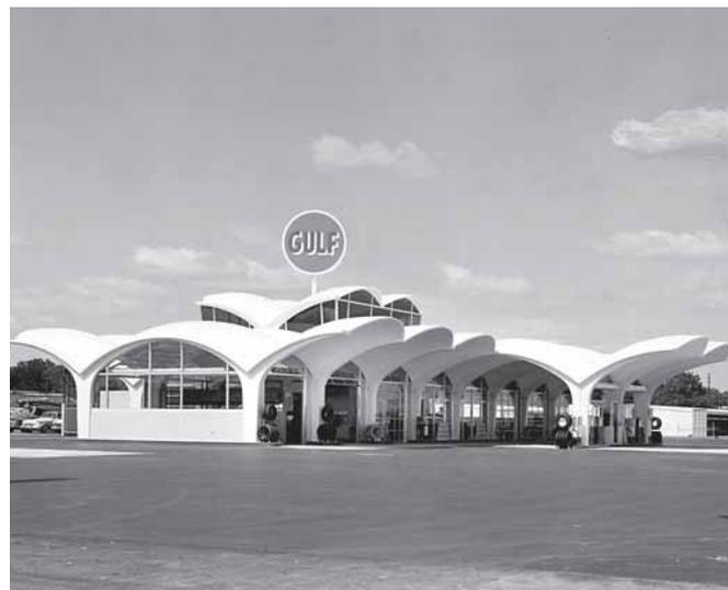
Concrete shell structures show up in everyday service. Left: Built around 1930, this was a Shell Oil Co. service station (now a repair shop) in Winston-Salem, NC. Although eight of these stations were built, this is the only one remaining and is now listed on the National Register. Right: A 1962 Gulf Oil Co. service station was much bigger and featured multiple shells in dramatic fashion. *ACI archives. Photos courtesy of JoAnn Sieburg-Baker (left) and Gulf Oil Co. (right).*
