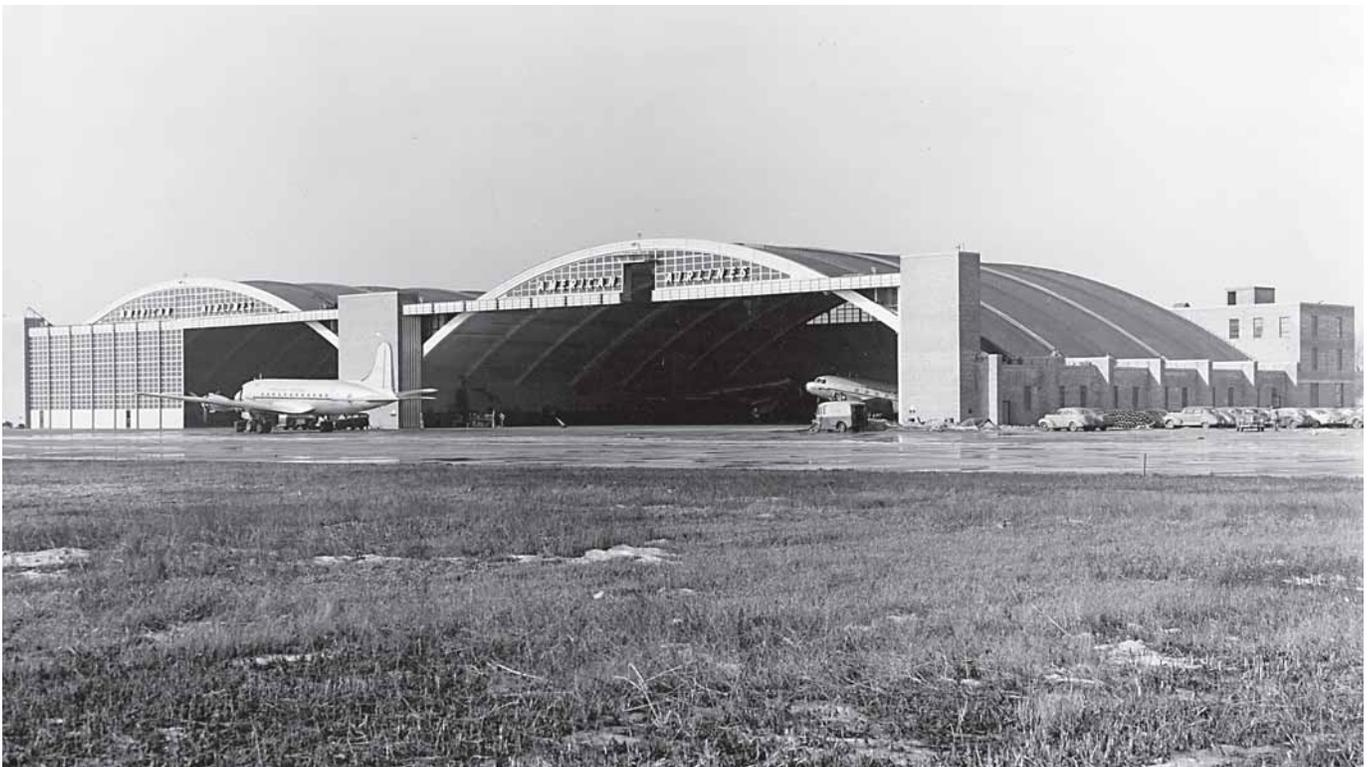
The reinforced concrete thin shell American Airlines hangar at Chicago's Midway Airport, built in 1947-1948, was one of the largest commercial airline hangars at the time; eight DC3s could be serviced in each hangar at one time. Each hangar had a clear span of 257 ft (78 m) with a rise of 42 ft (13 m).
