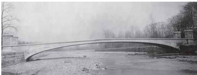
An early twentieth century project. A three-hinged concrete arch bridge in Brookside Park, Cleveland, OH, built by the Block Bridge & Culvert Co. of Indianapolis, IN.
