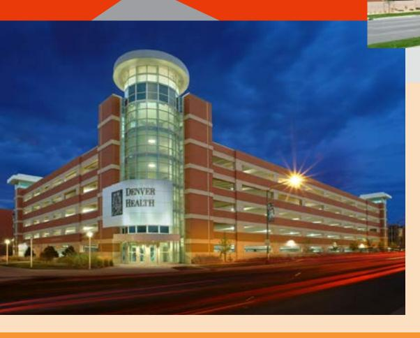
The Denver Health Employee Parking Garage provides 228,000 ft² of parking in five stories. The structure has an open interior created by double tees that span between "spread walls" and K-frames, which also resist lateral loads. Altogether, 927 pieces of architectural and structural precast products went into the building. The architectural concrete wall panels were cast with thin brick, and the surrounding colored concrete was lightly acid-etched.
