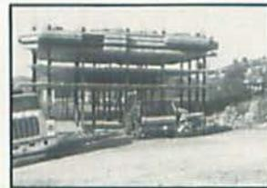
Lift Slab Construction: The best qualities of steel and concrete construction at an economical cost.
