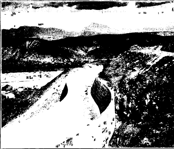
FIG. 4.—A PORTION OF THE CONCRETE-LINED POWER CANAL NEAR ROOSEVELT, ARIZONA.
