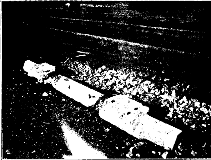
FIG. 8.—MANNER OF FAILURE OF REINFORCED CONCRETE TIES IN LONDON AND SOUTHEASTERN RAILWAY.
