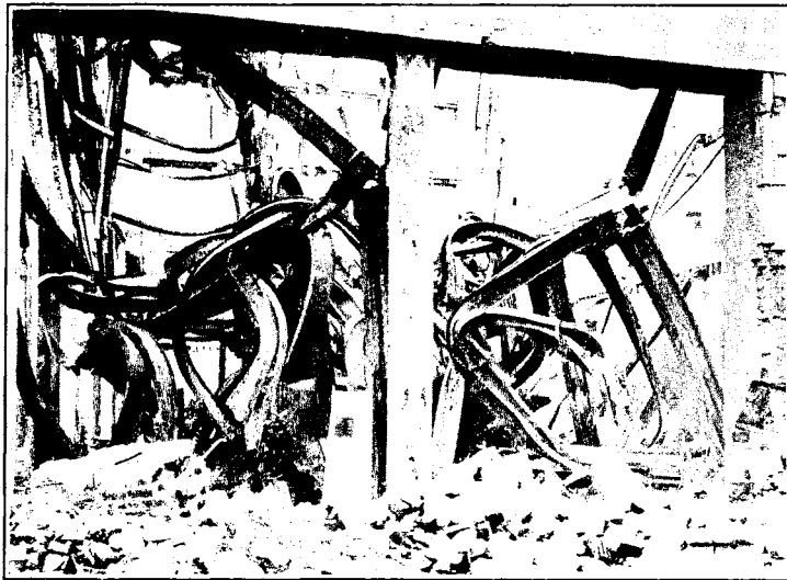
FIG. 13.—RESULT OF FIRE IN BUILDING WITH UNPROTECTED STEEL STRUCTURAL MEMBERS.
