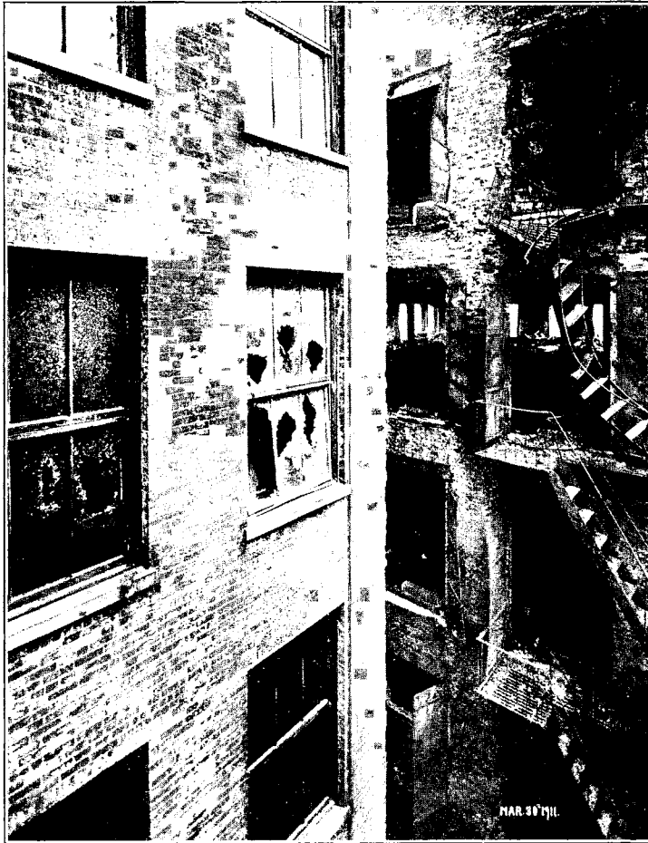
FIG. 4.—FIREPROOF BUILDING ADJACENT TO ASCH BUILDING, NEW YORK, SHOWING PROTECTION AFFORDED BY WIRE GLASS IN METAL FRAMES.
