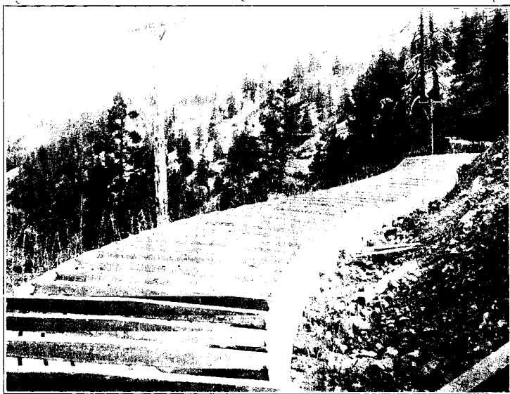
FIG. 6.—MAIN TIETON CANAL, YAKIMA PROJECT, WASHINGTON.
