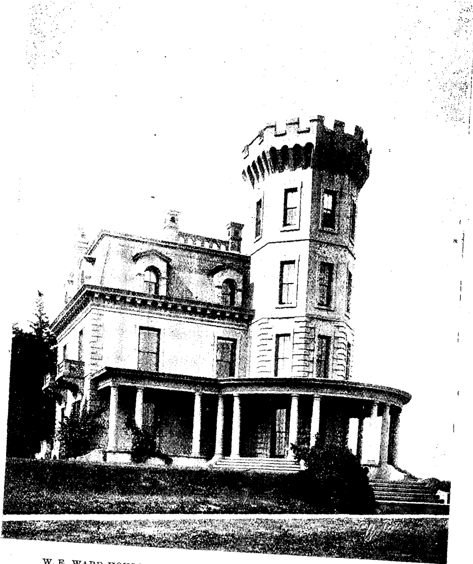
W. E. WARD HOUSE, CONCRETE SKELETON. BUILT 1875. NEW YORK.
