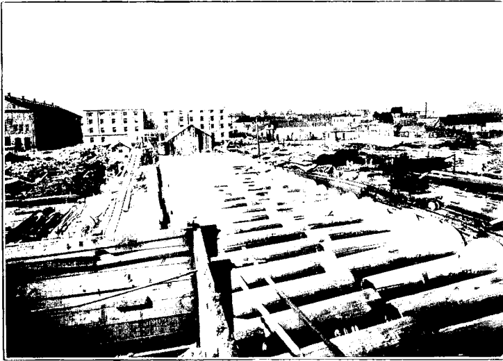
FIG. 12.—REINFORCED CONCRETE PILE SHELLS FOR PIER 8, NAVY YARD, PUGET SOUND, WASHINGTON.
