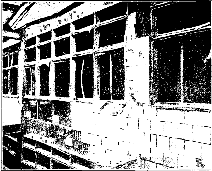
FIG. 5.—WELLS-FARGO BUILDING, SAN FRANCISCO, SHOWING EFFECT OF FIRE.
