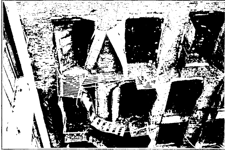
FIG. 40.—FIRE ESCAPES, ASCH BUILDING, NEW YORK, N. Y.
