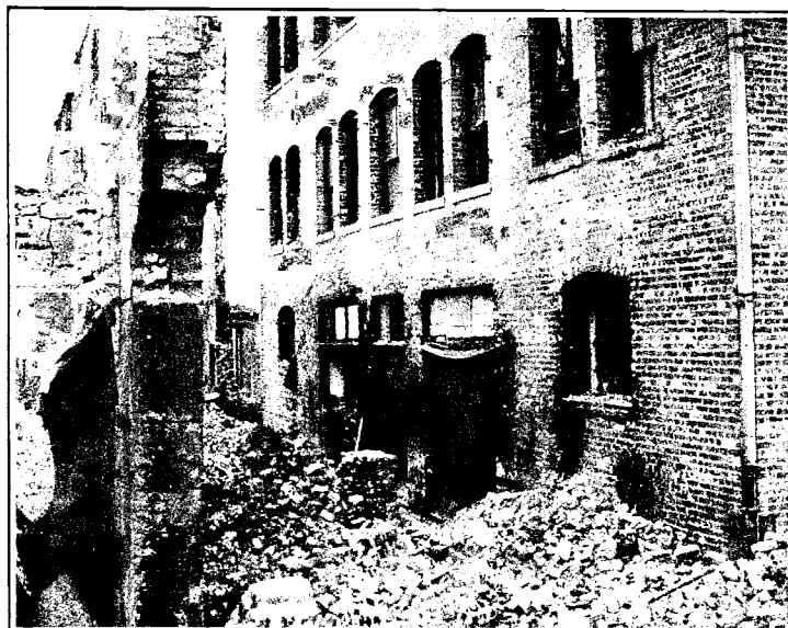
FIG. 6.—VOLKMAN BUILDING, SHOWING PROTECTION AFFORDED BY FIREPROOF DOORS AND WINDOWS.
