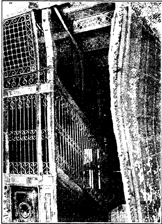
FIG. 30.—FAILURE OF PARTITION OF PLASTERED METAL FABRIC SUPPORTED BY ANGLE IRONS.
