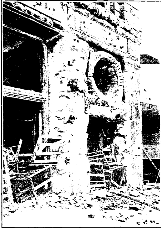
FIG. 8.—ORNAMENTAL STONE WORK DAMAGED BY FIRE, ENTRANCE TO E.TNA BUILDING, SAN FRANCISCO.
