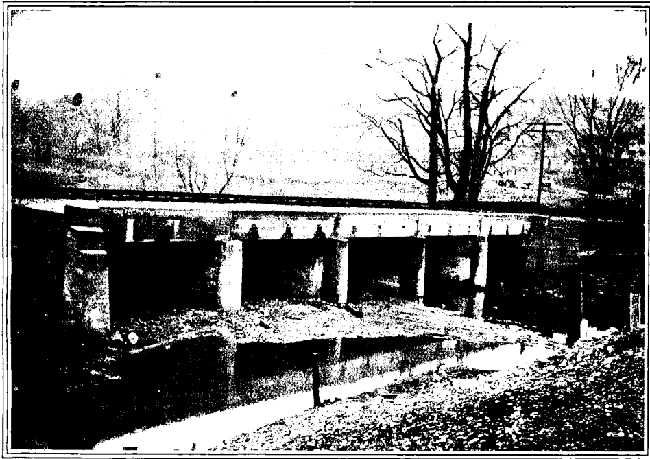
REINFORCED CONCRETE TRESTLE ON LINE BURLINGTON RAILROAD.
