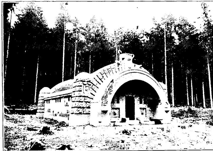
FIG. 17.—REINFORCED CONCRETE ENTRANCE TO SHAFT, WATER WORKS AT BEYREUTH, GERMANY.
