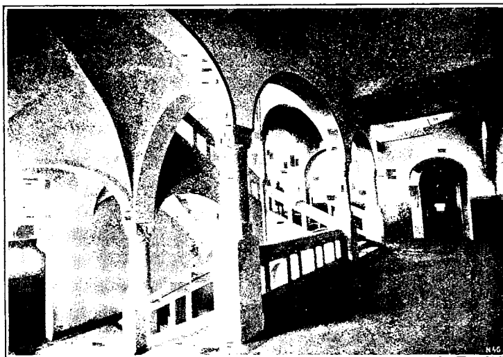
FIG. 24.—REINFORCED CONCRETE STAIRWAY, NORTH SCHOOL, JENA, GERMANY.
