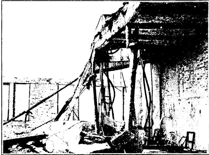
FIG. 12.—FAILURE OF CAST IRON COLUMNS, CAUSING COLLAPSE OF CINDER CONCRETE FLOOR.
