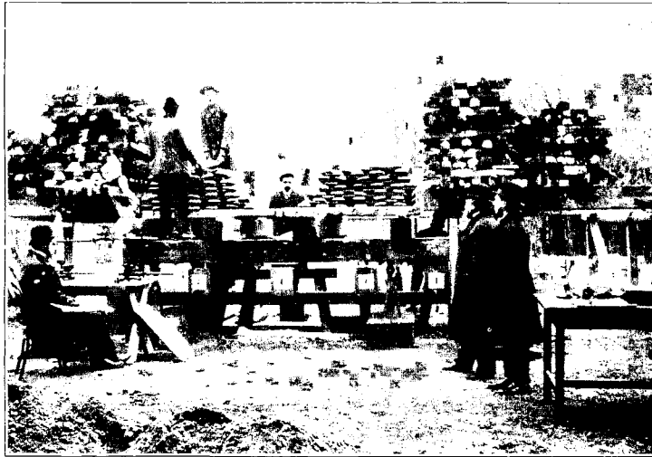
FIG. 23.—METHOD OF APPLYING LOAD IN TESTING REINFORCED CONCRETE BEAMS.
