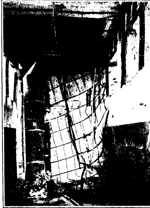
FIG. 35.—FAILURE OF SUSPENDED CEILING.
