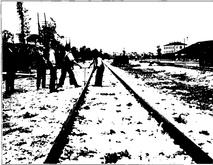
FIG. 6.—REINFORCED CONCRETE TIES IN MAIN LINE ITALIAN RAILWAY AT PORTO NACCIO, ITALY.
