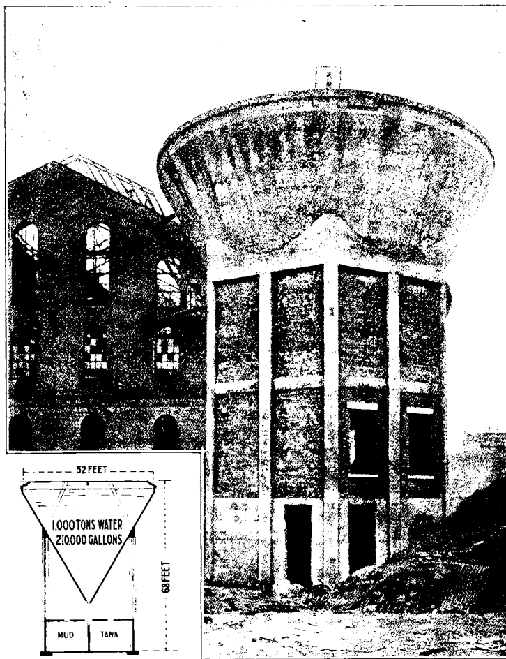
FIG. 14.—REINFORCED CONCRETE SETTLING TANK, SILVERWOOD COLLIERIES, ROTHERHAM, ENGLAND.
