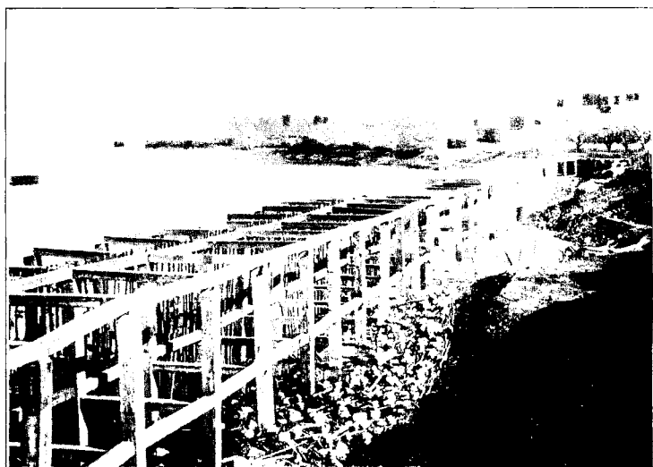
FIG. 11.—REINFORCED CONCRETE DIKE AT ST. JOSEPH, MISSOURI.
