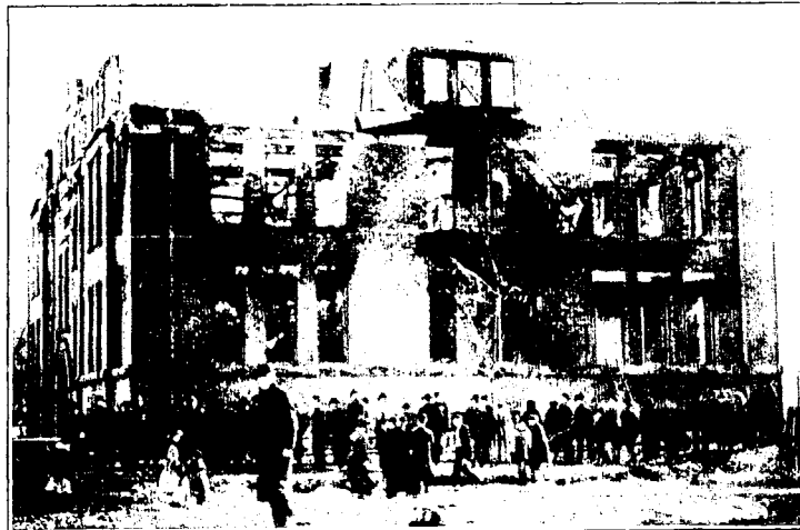
FIG. 41.—FIRE ESCAPES, SCHOOL BUILDING, COLLINGSWOOD, OHIO.
