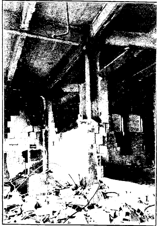
FIG. 31.—FAILURE OF TERRA COTTA PARTITION.
