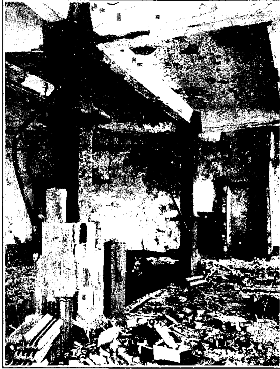
FIG. 20.—FAILURE OF STEEL COLUMN THROUGH EXPANSION OF ENCLOSED PIPES DESTROYING THE TERRA COTTA FIREPROOFING.
