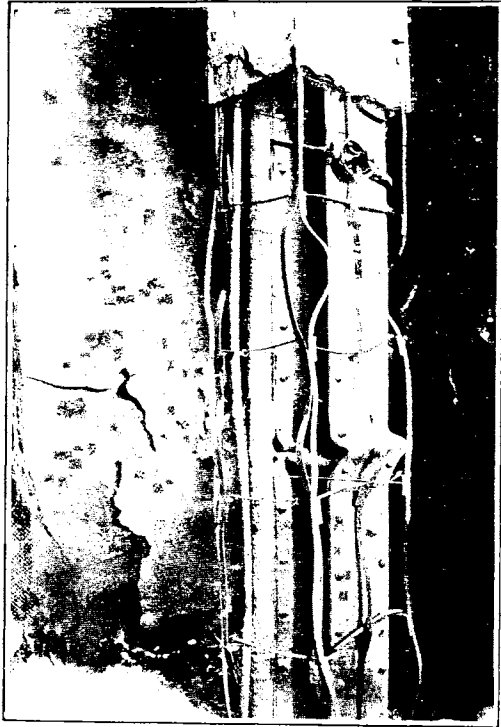
FIG. 17.—FAILURE OF COLUMN PROTECTED BY SINGLE LAYER OF WOVEN WIRE COVERED WITH HARD PLASTER.
