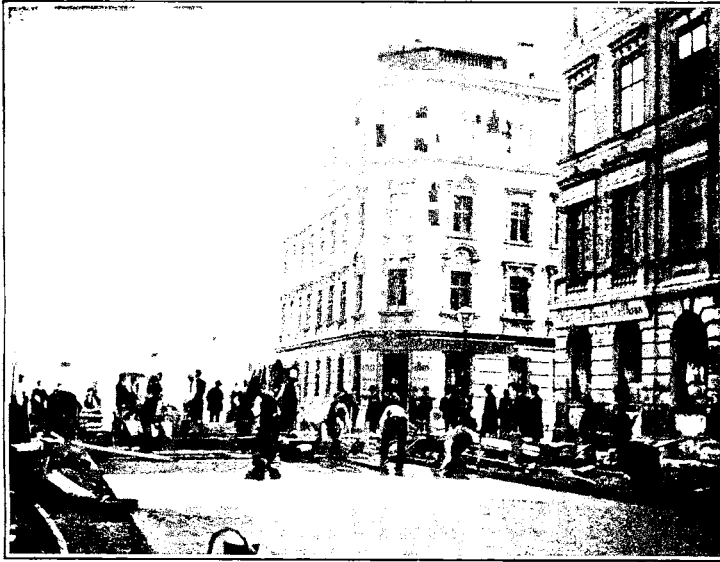
FIG 10.—CONCRETE PAVEMENT UNDER CONSTRUCTION IN HASNER STREET, VIENNA, AUSTRIA.
