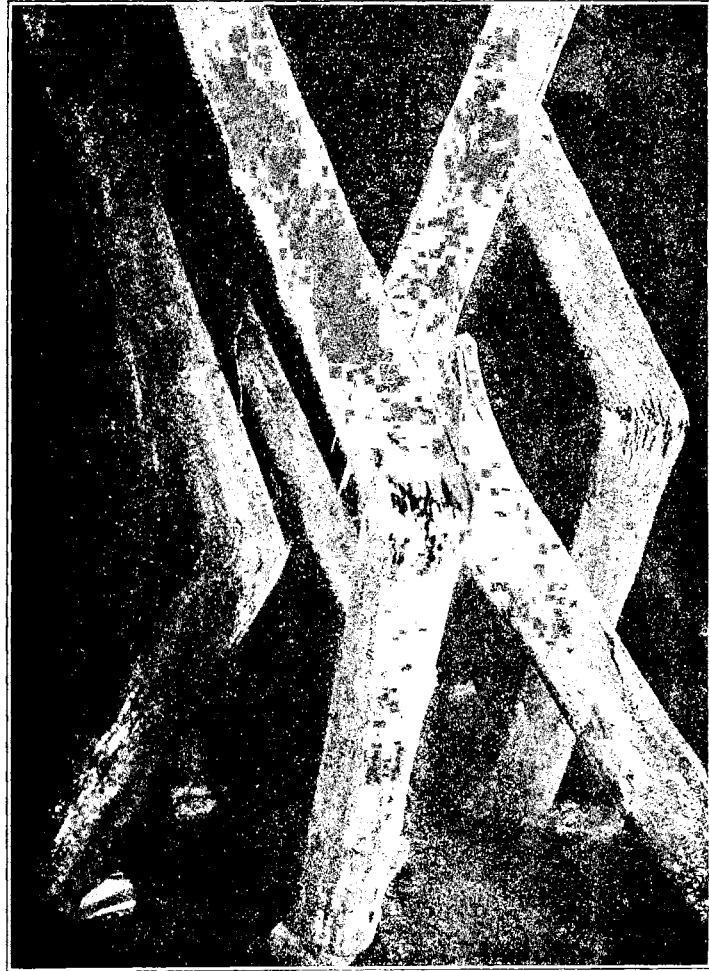
FIG. 9.—MANNER OF FAILURE OF WOODEN MINE PROPS.
