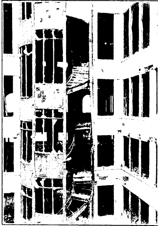
FIG. 42.—FAILURE OF POORLY PROTECTED STAIRWAY.
