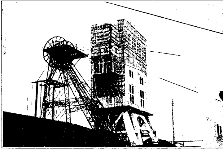
FIG. 10.—REINFORCED CONCRETE HEAD HOUSE AT CAMPHAUSEN, GERMANY.
