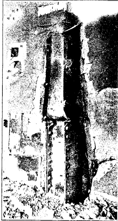
FIG. 16.—BUCKLED COLUMN, HOTEL HAMILTON, SAN FRANCISCO.
