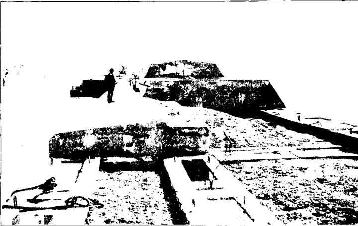
FIG. 10.—BREAKWATER AT BUFFALO, N. Y., SHOWING MANNER OF CONSTRUCTION.
