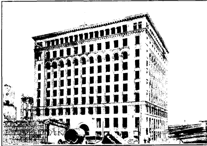
FIG. 1.—MILLS BUILDING, SAN FRANCISCO, AFTER FIRE.
