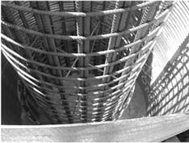
Fig. 2.2.2(c)—Hoop reinforcement in a reinforced concrete column (courtesy of HDR Engineering, Inc.).
