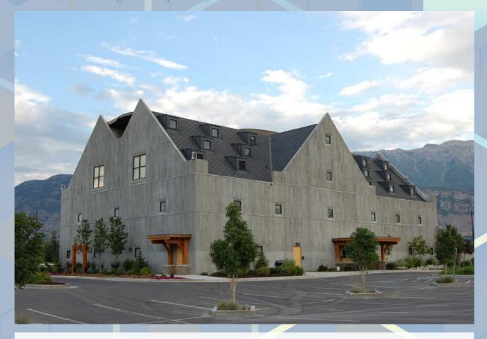
What is more exciting, the virtual reality games taking place inside or the fact that this unique building is made out of precast concrete? Board-finish form liners were used to create a wood-like exterior finish on insulated structural precast panels.
