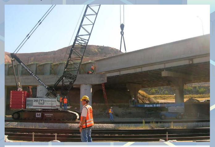
The overpass was the first UDOT bridge to meet the seismic design designation of "operational," meaning that the bridge must remain functional in the event of an earthquake. The bridge is made up of 92 precast concrete girders. Some girders span 198 ft (60 m) to minimize disruptions to the trains below and the vehicles above. Precast elements also included partial-depth panels for the composite bridge deck.
