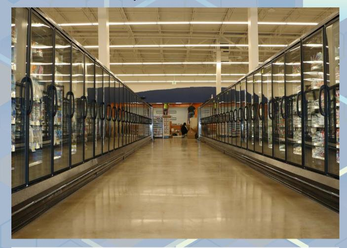
Kent's Market used the patented concrete system MagicSlab™, which eliminates joints and reduces cracks and visible saw-cuts. The market floor used a single placement of 34,000 ft² (3160 m²) of this concrete slab and eliminated more than 9000 ft (2740 m) of saw-cut joints.
