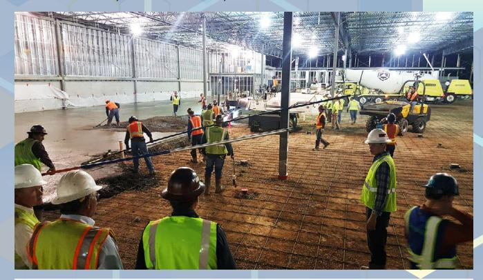
The 60,000 yd³ (45,870 m³) placement for the supermarket slab prompted an aggressive plan for a 1-day operation that broke company records. The slab placement required 98 concrete trucks, four crews of over 60 workers, and 28 hours—all of which saved 2 weeks on the schedule. The cost to bring in crews from across the country was more than recovered in saved labor costs. More important was the chance to have employees from across the company work together and spend time catching up.
