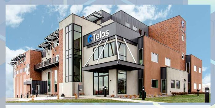
Telos U is a five-story, 74,000 ft² (6870 m²) architectural tilt-up concrete structure, with two stories of living space atop a three-story gymnasium. The 60 ft (18 m) tall tilt-up panels incorporate integrally colored concrete and thin-brick accents, resulting in rich coloring and texture. Because the design called for exposed polished concrete floors, special care and consideration needed to be taken not to damage the casting floor while handling the enormous panels.
