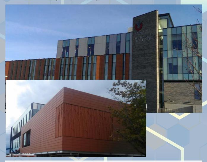
The school features unique decorative glass fiber-reinforced concrete (GFRC) panels as a focal point at the front of the building, using a red color in the GFRC to match terracotta panels in other areas. The pattern cast into the panels using a custom rubber mold has the look of tree trunks and branches with a background of desert cracked clay bed. The panels were integrated with a continuous insulation system to achieve a sustainable design complementing the beauty of the building.
