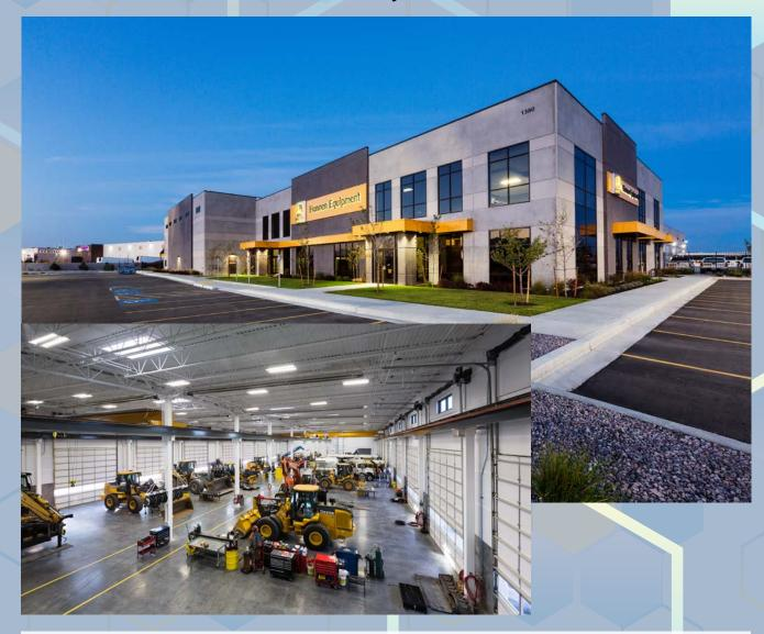
Honnen Equipment is a tilt-up concrete office and warehouse building, designed for the sales and service of heavy earth-moving equipment. The exterior exposed concrete walls use both natural and "black" concrete. Some of the surfaces are also partially sandblasted, creating subtle stripes. Post-tensioning was used on the floor slab to minimize the number of control joints, and colored concrete was used for the polished finish.
