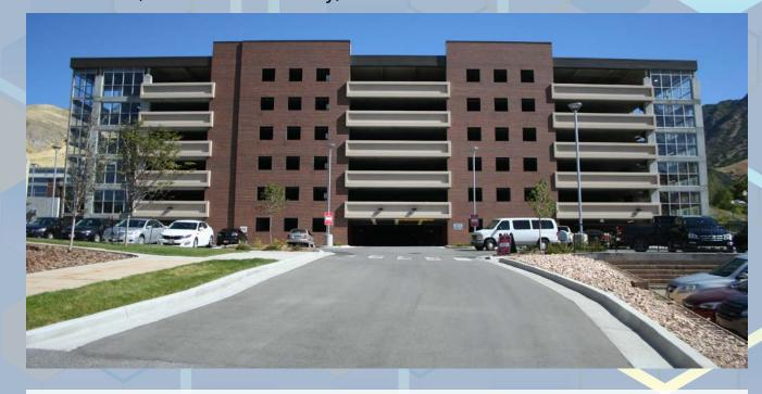
This six-level, concrete-based garage uses a precast concrete panel and masonry exterior, making it aesthetically pleasing and space efficient. The exposed concrete on the garage's interior complements the precast concrete panels, masonry, and stainless steel exterior. The sloped-site project includes a cast-in-place retaining wall with an architectural finish.
