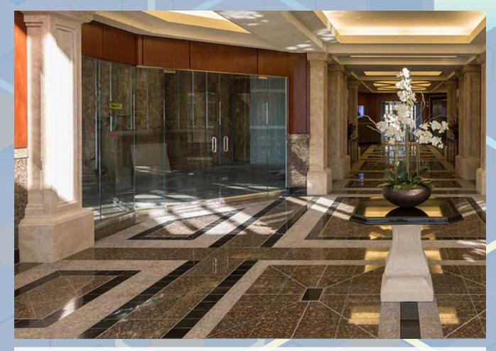
Thanksgiving Point office towers is a 22,000 ft² (2040 m²), mixed-used building with the third floor set aside for executive office suites near I-15, with quick access to many restaurants and hotels. Glass fiber-reinforced concrete (GFRC) column covers are located throughout the interior and exterior. The GFRC has a high-end, hen-picked finish to match natural stone. The GFRC and the high-quality woodwork in the lobby impart eloquence and class.
