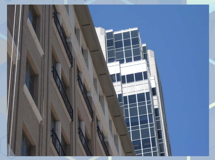
City Creek Center is a mixed-use development near Temple Square with an upscale, open-air shopping center; office and residential buildings; fountain; and simulated creek. Precast and glass fiber-reinforced concrete (GFRC) for the exterior façade of this six-story, 35,000 ft<sup>2</sup> (3250 m<sup>2</sup>) building include spandrel panels at the base of each window, window surrounds, cornices, and caps, and a top band of GFRC corbels and cornices.
