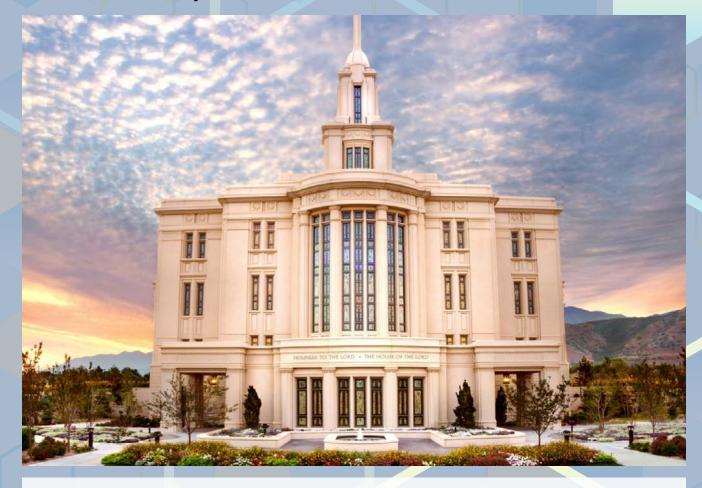
To achieve a high level of ornate detail and quality, precast concrete is consistently used to build stunning temples across the United States. This temple is no exception. Aggregate was imported from California and panels were sandblasted to achieve the exact finish desired. The precast roof and wall panels cover a steel frame structure, increasing the speed of enclosure after the supporting structure is in place.
