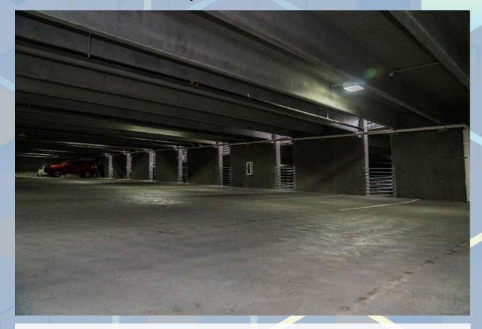
This five-level parking garage sits at the core of the Alta Gateway Station Apartments, which wrap around the garage, hiding it, and allowing residents to park on the same level as their residence. The garage uses precast, prestressed double tees. Their long spans resulted in needing only two precast columns inside the entire garage, maximizing the number of parking spaces. Precast shear walls, each five levels tall, are spaced strategically to allow visibility and light between floors.
