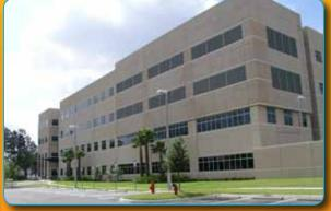
state-of-the-art treatment and research facility, M2Gen is the result of a partnership between Moffitt and drug maker Merck & Co. The exterior features three-colored architectural precast concrete in 247 panels covering 36,600 ft². The chemically retarded exposed aggregate finish was expressed with a medium abrasive blast. Architect: Reynolds, Smith & Hills, Inc. Contractor: Skanska USA.
