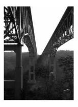
at 2230 ft. The bridge is currently undergoing a complete reconstruction, with the existing twin steel bridges being replaced with twin cast-in-place concrete segmental box structures using the balanced cantilever method of construction. This tour will give you an inside look at the construction of the replacement structures that cross a National Scenic River and Valley.
