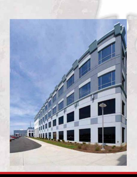
This LEED Gold project involved two four-story office buildings designed with tilt-up concrete exterior walls and concrete floor slabs. The tilt-up panels were crucial to the building's aesthetic and to the project's sustainability, providing long life with minimum maintenance. The development brought 1700 employees to the region, boosting the economic vitality of the West Chester Community.
