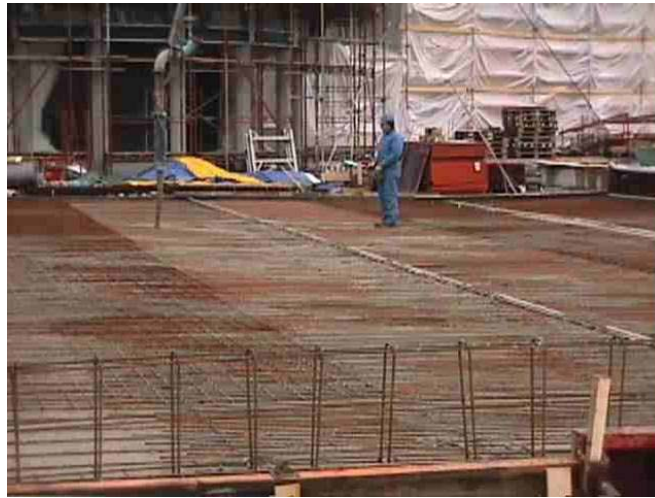
Fig. 1 - Casting of SCC in a one-man operation (Courtesy of NCC Sweden).
