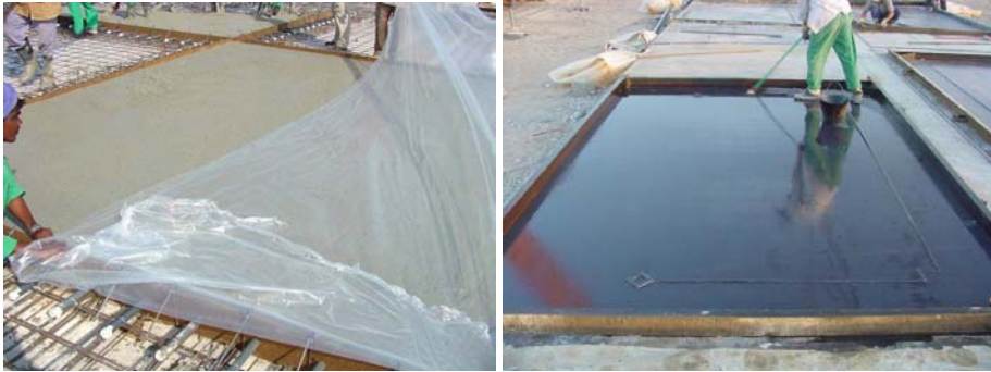
Fig 12 - Good curing practice has to be applied also for SCC (Courtesy of M. Sonebi)
