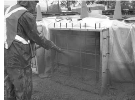
Fig. 8.8—Bench shooting thick preconstruction panel.
