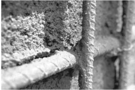
Fig. 8.13—Another quality application. Note even build-out of material and how ridge has been formed in it.
