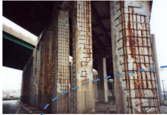
(Vector Corrosion Technologies)
