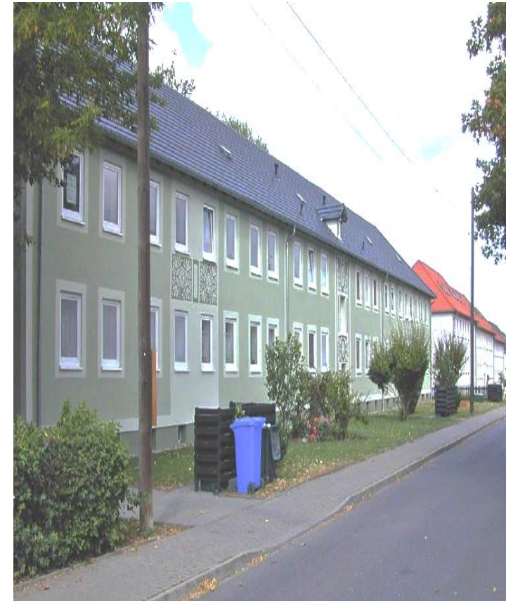
Multi-family apartment building using rammed earth in Mücheln, Germany (1955)
