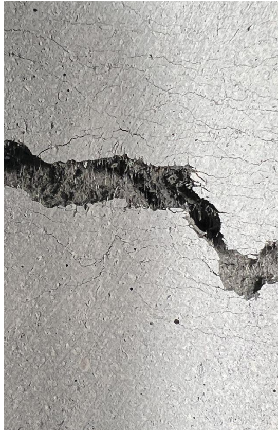
Engineered Cementitious Composites (ECC)
