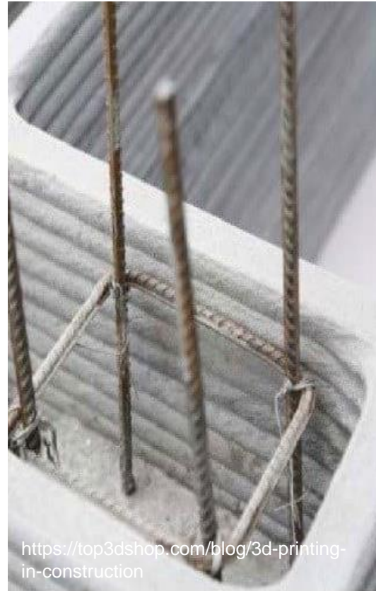
Pre-installed reinforcement
