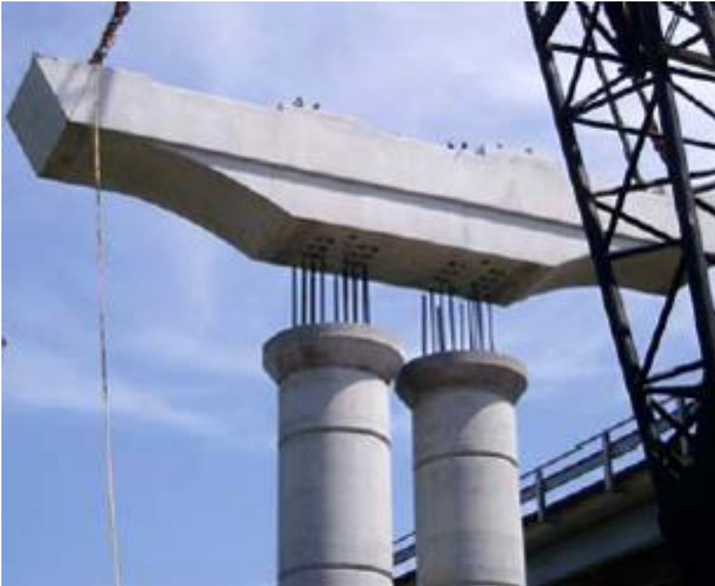
Lake Belton Bridge Replacement (FHWA, 2009)
