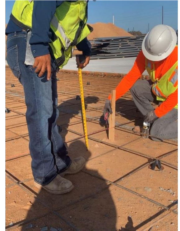
Checking subgrade elevation with string line and tape measure
