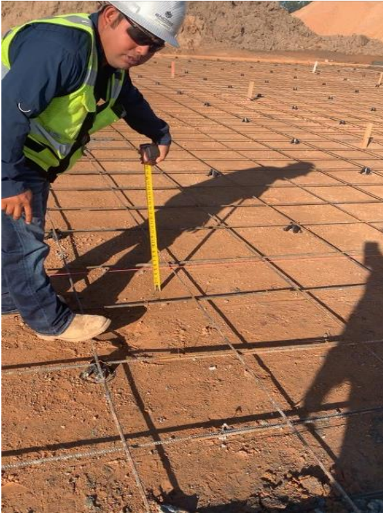
Checking subgrade elevation with string line and tape measure
