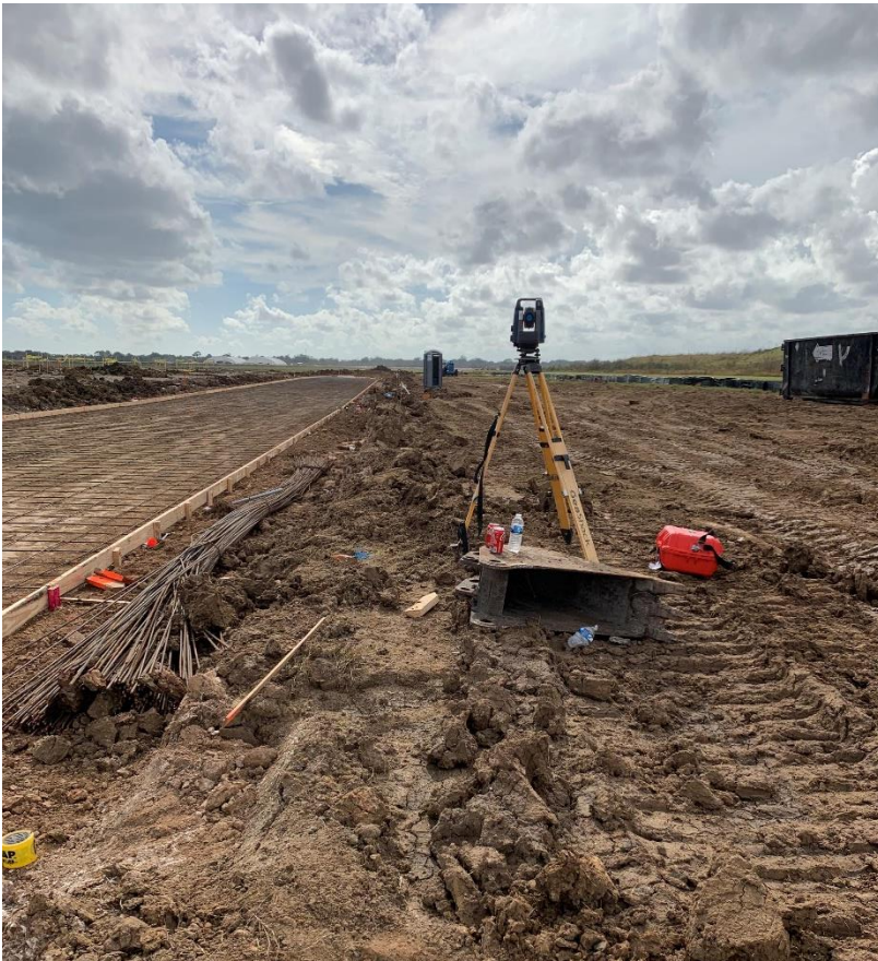
Total station set up
