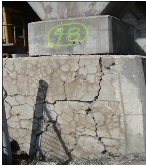
Source: "Condition assessment of an ASR-affected overpass after nearly 50 years in service," Sanchez et al., Construction and Building Materials , 2018.
