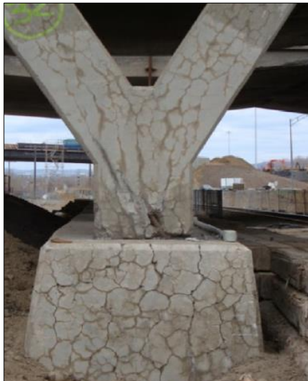
Source: "Condition assessment of an ASR-affected overpass after nearly 50 years in service," Sanchez et al., Construction and Building Materials , 2018.
