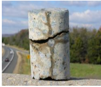
C5 - delamination at 2.5 inches
