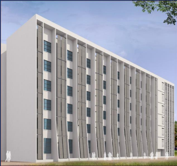
Inclined Fin Walls (Form Finish)
