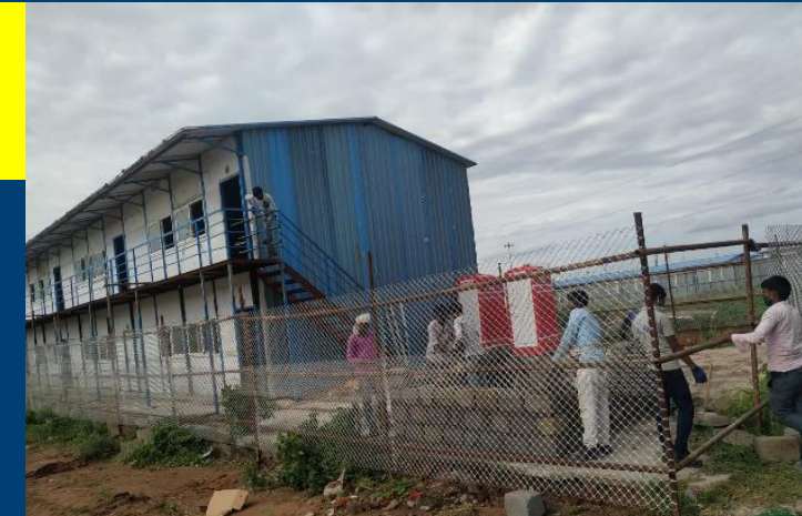
Isolation Wards at Workmen Colony
