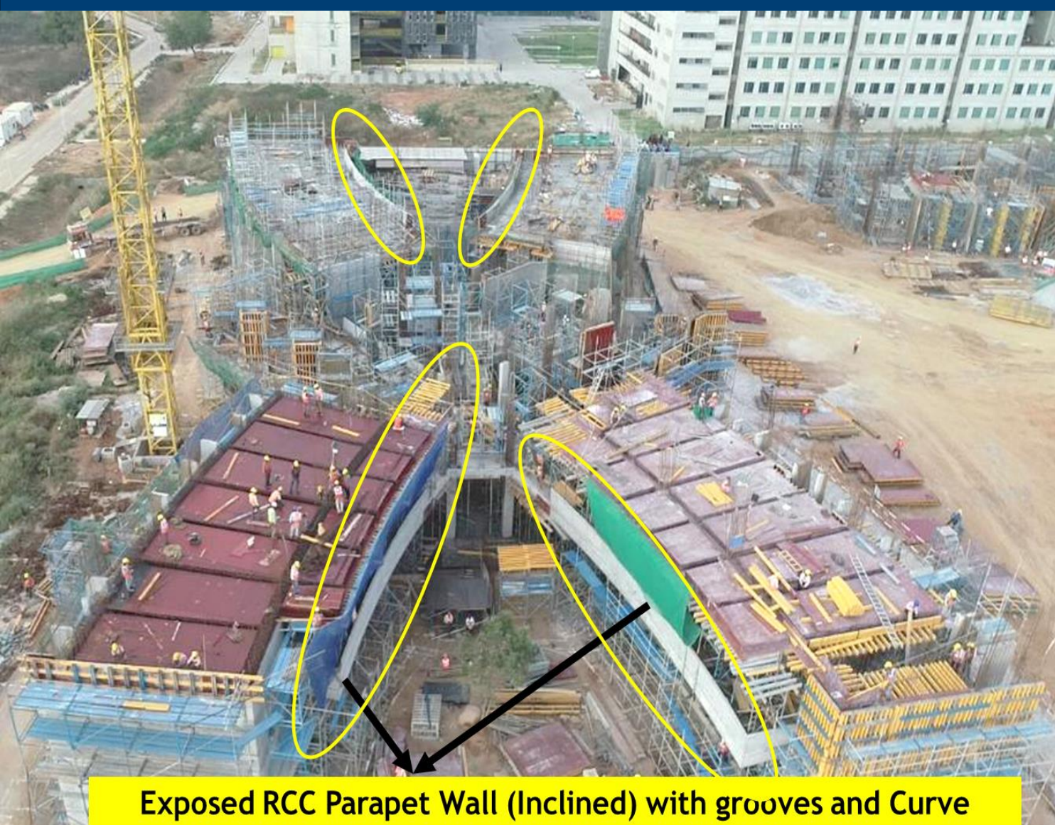
Exposed RCC Wall (Inclined & Curved) with grooves
