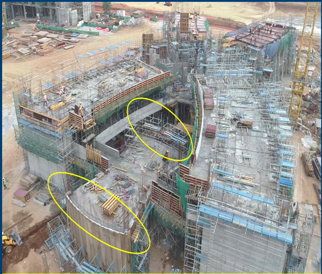
Exposed RCC Wall (Inclined & Curved) with grooves
