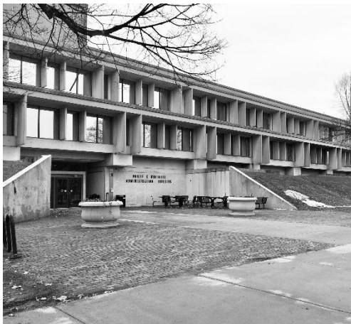
Whitmore Administration Building Campbell & Alrich, 1967
