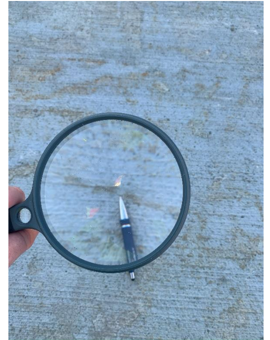
Shrinkage Cracking
