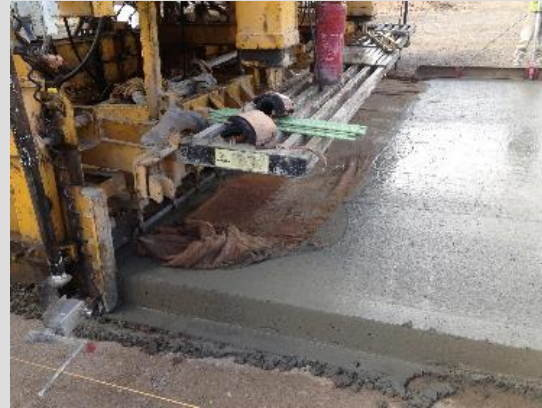
Placement of Concrete with Nano Silica
