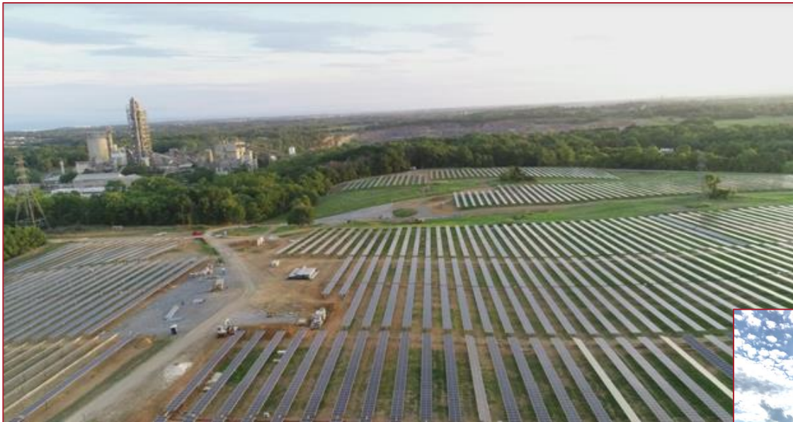
Solar Panels at Hagerstown, MD
