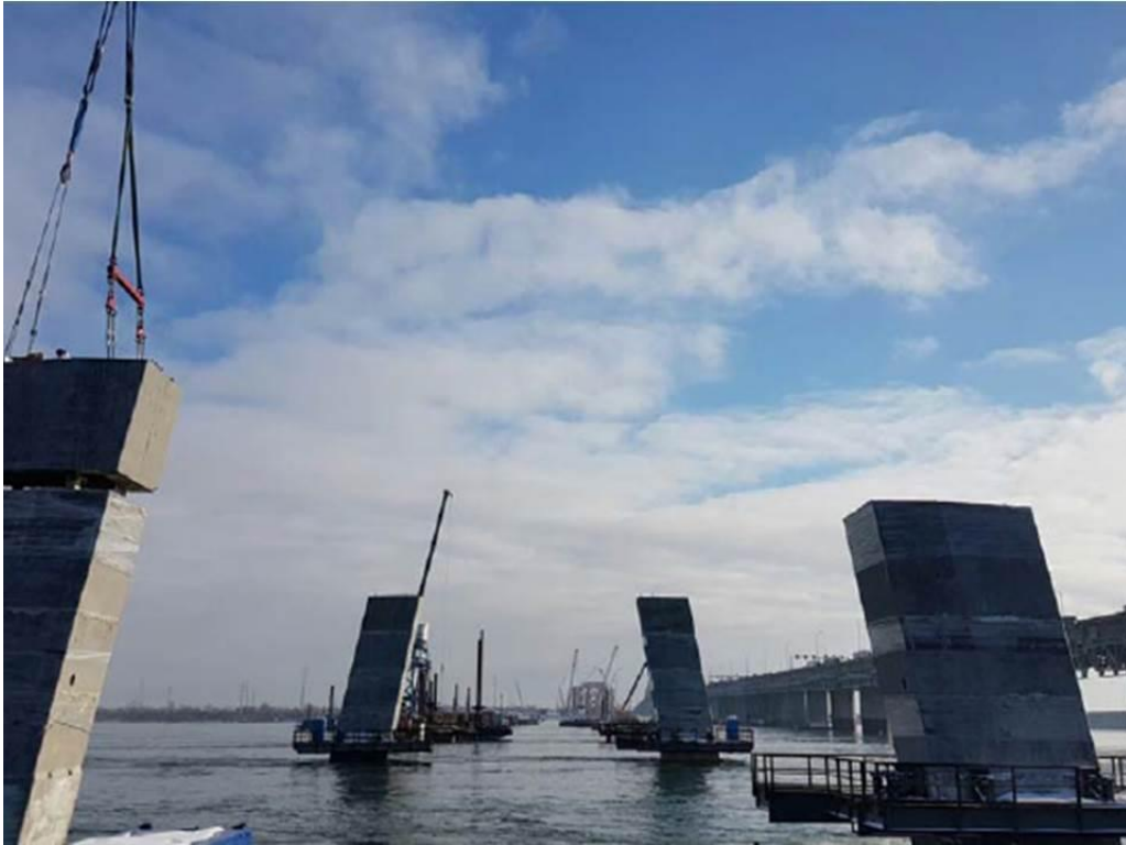
Construction Photo: October 2016
