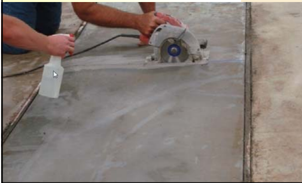
1 in. Saw-Cut Joints Cut at 24 hours
