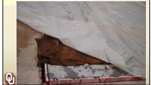
7 Day Curing Concrete with Wet Burlap & Plastic Sheet
