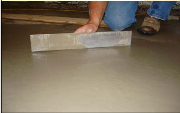
Finishing Concrete
