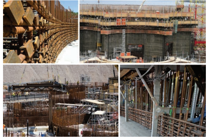
Fig. 9: Slipforming of walls with high-density reinforcement helped to minimize schedule and improve leak-tightness by eliminating most construction joints
