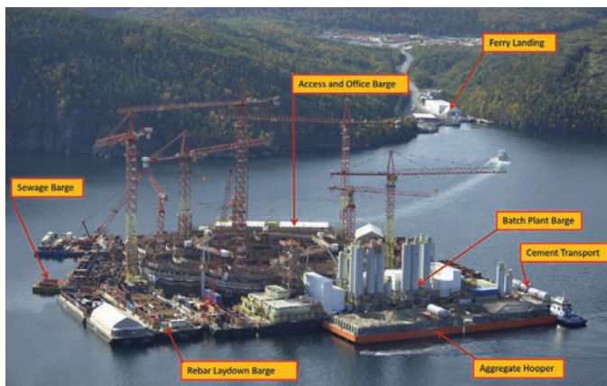
Fig. 10: Construction at deep-water site required 12 support barges stationed around the GBS
