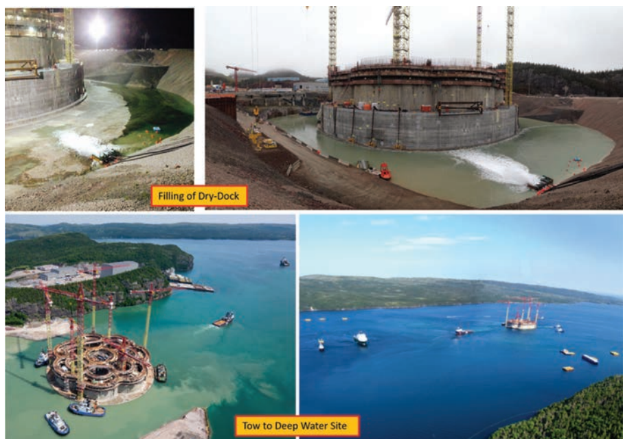
Fig. 4: After filling of the dry dock with water, the GBS was towed to the deep water site
