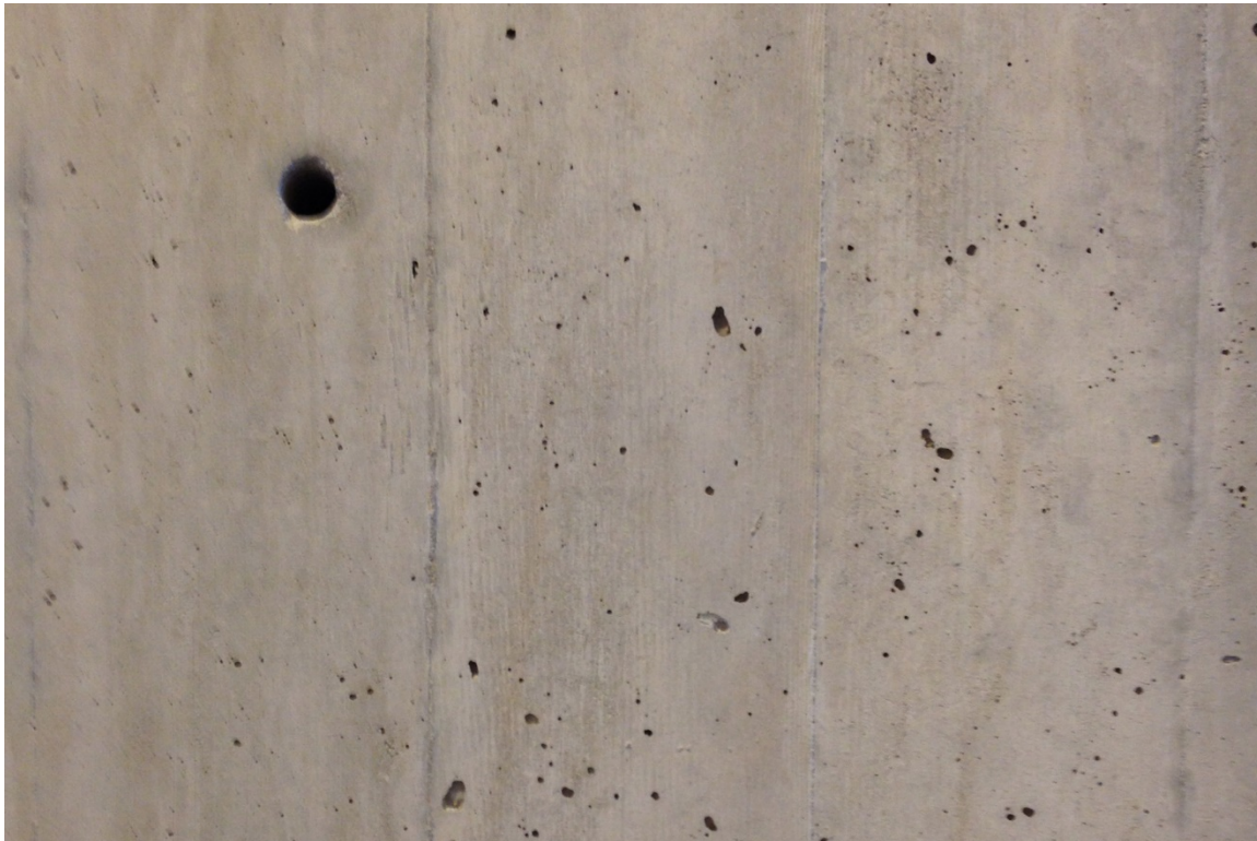
Fig. 4 Photos of board-finished walls in an award-winning museum. Note the number and size of bugholes, which were considered by a panel of architects to be a pleasant aesthetic feature of the museum's interior. (Photos courtesy of the Herbert F. Johnson Museum of Art, Cornell University)
