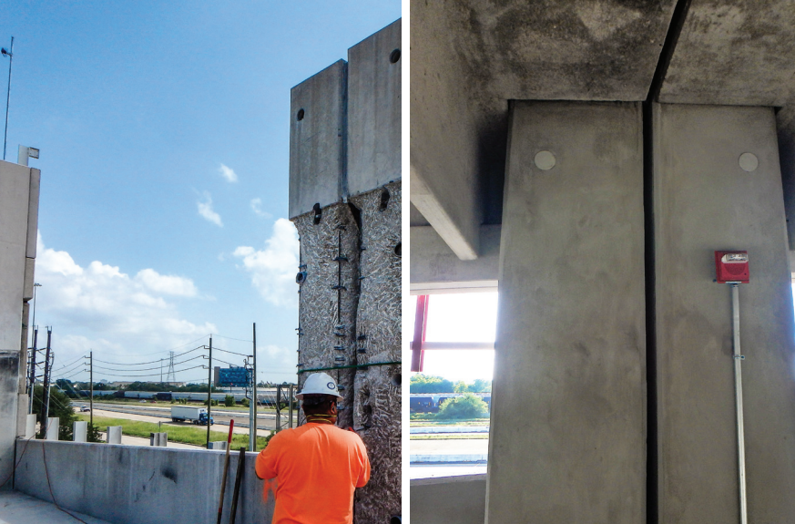
Fig. 9—Column during repair (left) and after repair (right)
