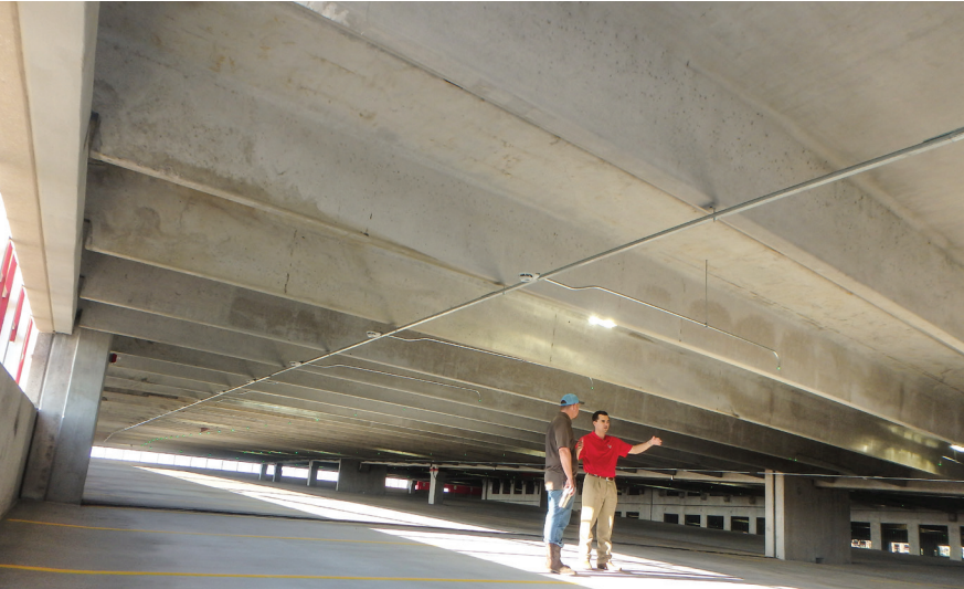
Fig. 8—New replacement double-tee beams at completion
