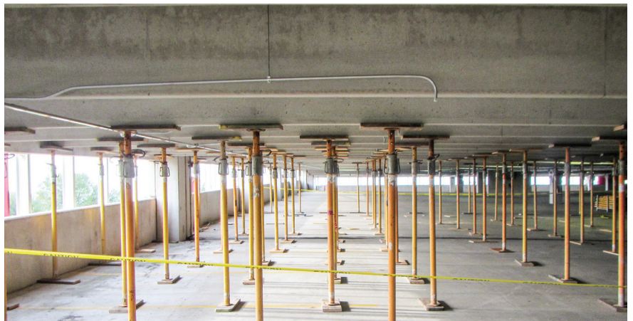
Fig. 4—Shoring installed in affected areas
