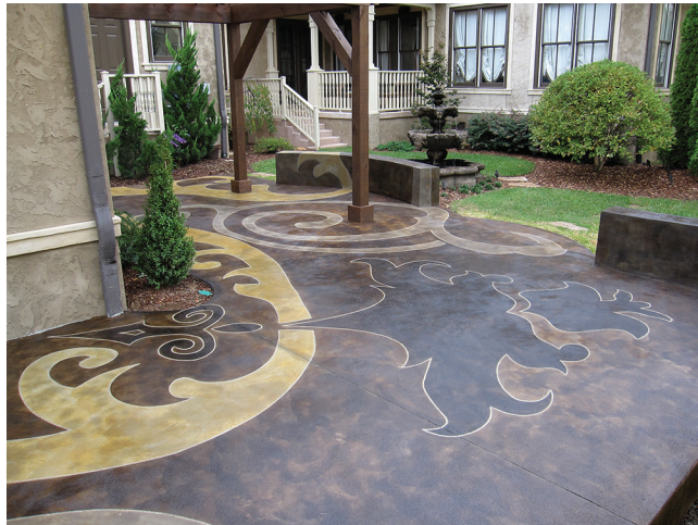
Fig. 1.2a—Cast-in-place decorative concrete combining treatments during and post placement to achieve aesthetic effects (courtesy of Concrete Mystique Engraving).
