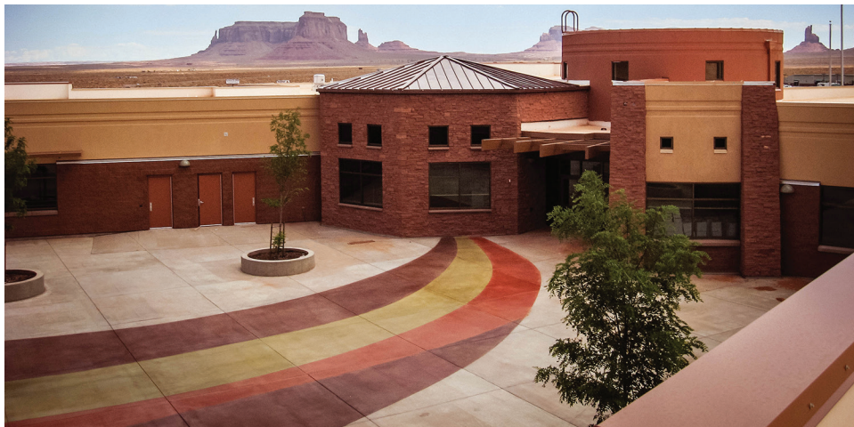
Fig. 1.2b—Decorative concrete applications such as post placement colorants can complement or enhance the overall aesthetics of a project (courtesy of PROSOCO).
