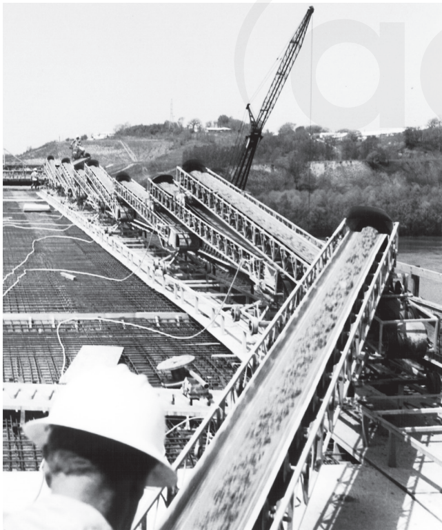
Fig. 4.5b—Feeder conveyors supplying side-discharge conveyor on bridge deck.
