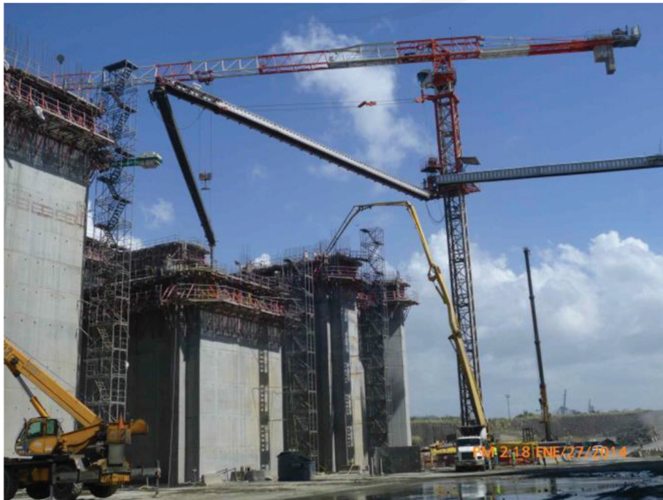
Fig. 4.4.1b—Cranes suspending conveyors to reach difficult access points.
