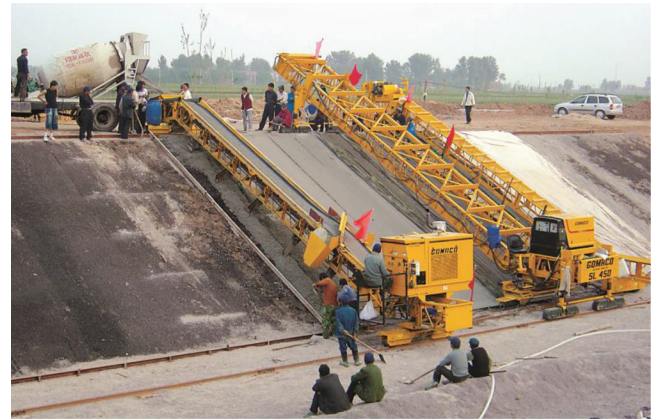
Fig. 4.4.2b—Side-discharge conveyor spreading concrete for slope placements.
