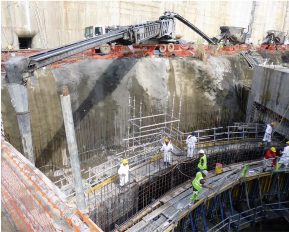
Fig. 4.5a—Portable conveyor supplying side-discharge concrete on elevated slab.
