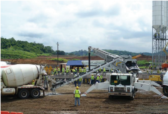
Fig. 4.4.1a—Radial spreading.
