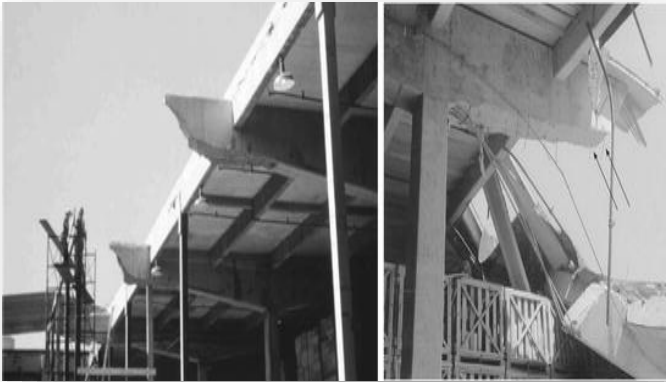
Shear Failure Wilkins Warehouse
