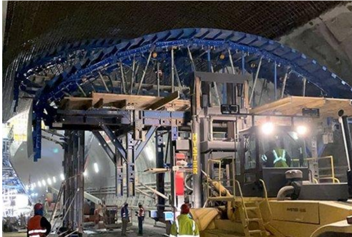
CAST IN PLACE
