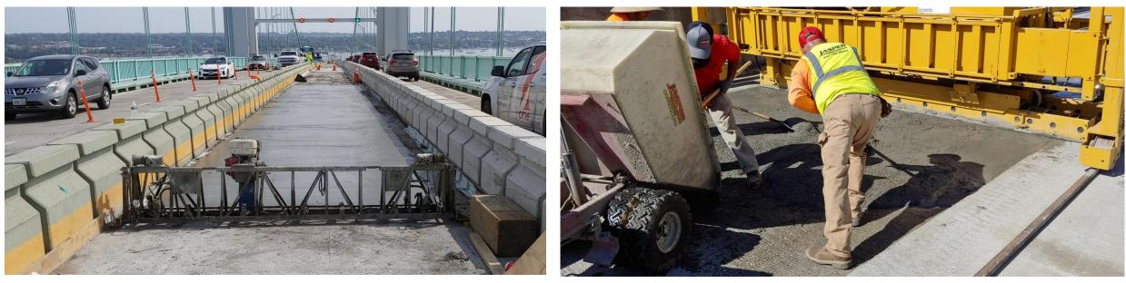
Placing the UHPC Overlay with a Vibrating Bridge Deck Truss Screed.
