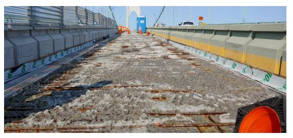
Finished Surface after Hydro-Demolition of the Claiborne Pell Newport Suspension Bridge, RI
