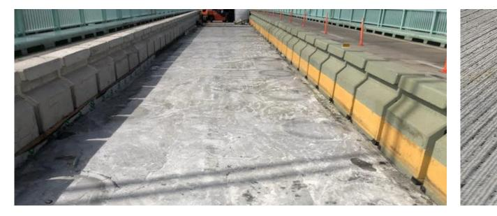
Finished & Cured UHPC Overlay surface prior to Grinding & Grooving.
