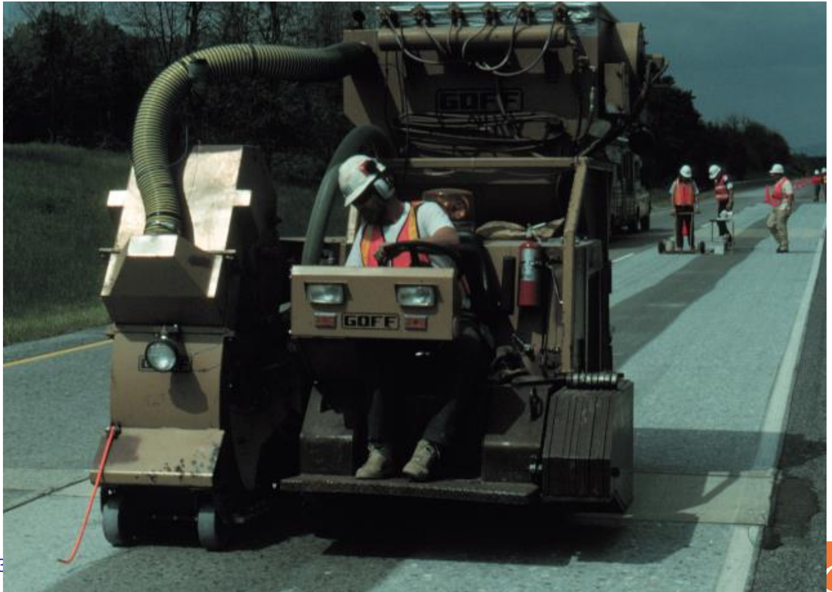
Fig 7, Abrasive shot-blasting
