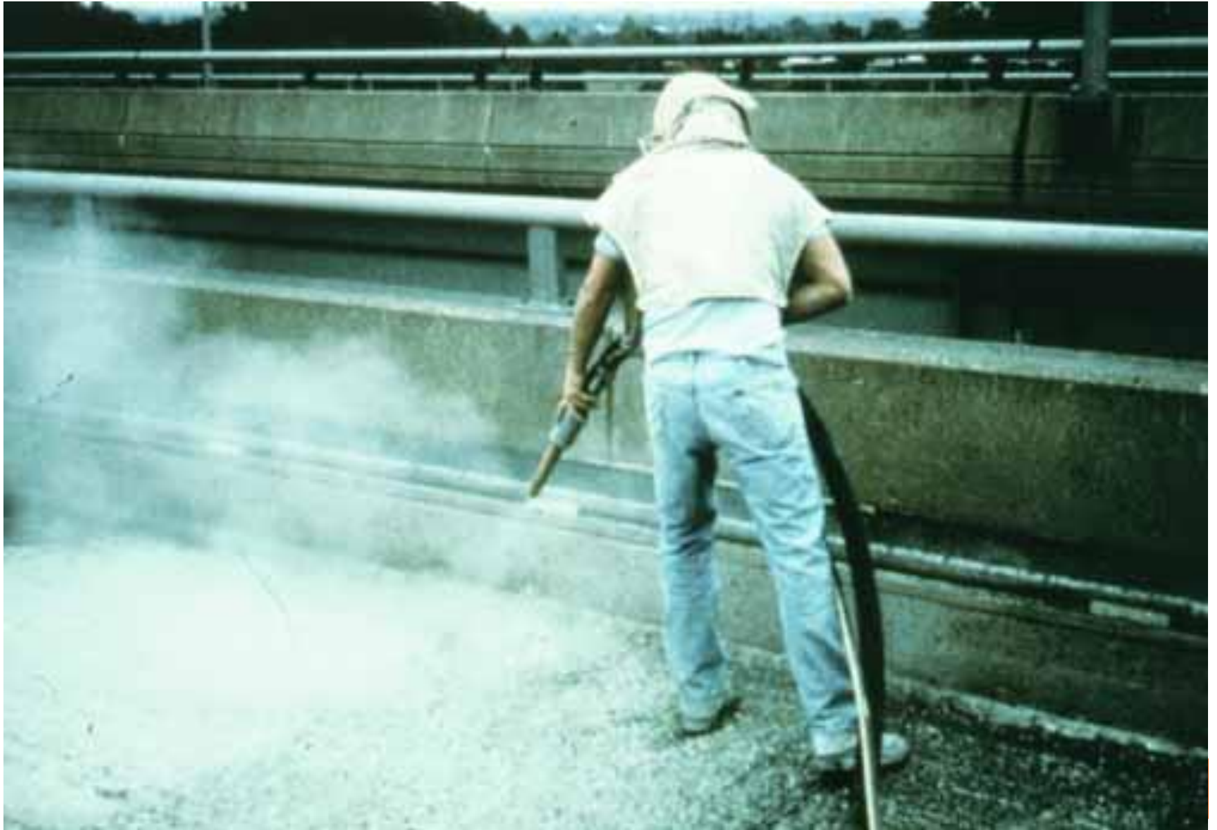
Fig 6, Abrasive blasting
